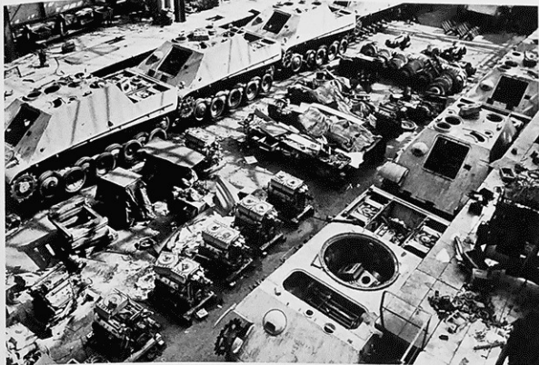
Above: The Maschinenfabrik Niedersachsen-Hanover was the only assembly firm that built Panthers and Jagdpanthers in series at the same time. The picture shows the chassis of a Type G Panther at the lower right; all those in back are Jagdpanthers. Between the two lines are engines ready for installation. Below: Two Jagdpanther bodies in the midst of Panther tank bodies, in production at MNH in April 1945.
