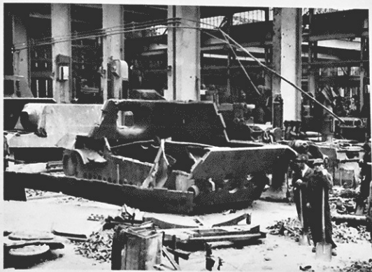
The Nibelungenwerk was hit by 143-ton explosive bombs during an Allied air raid on 10/16/1944. The considerable damage to the heavily armored Jagdtiger bodies came as a surprise.
