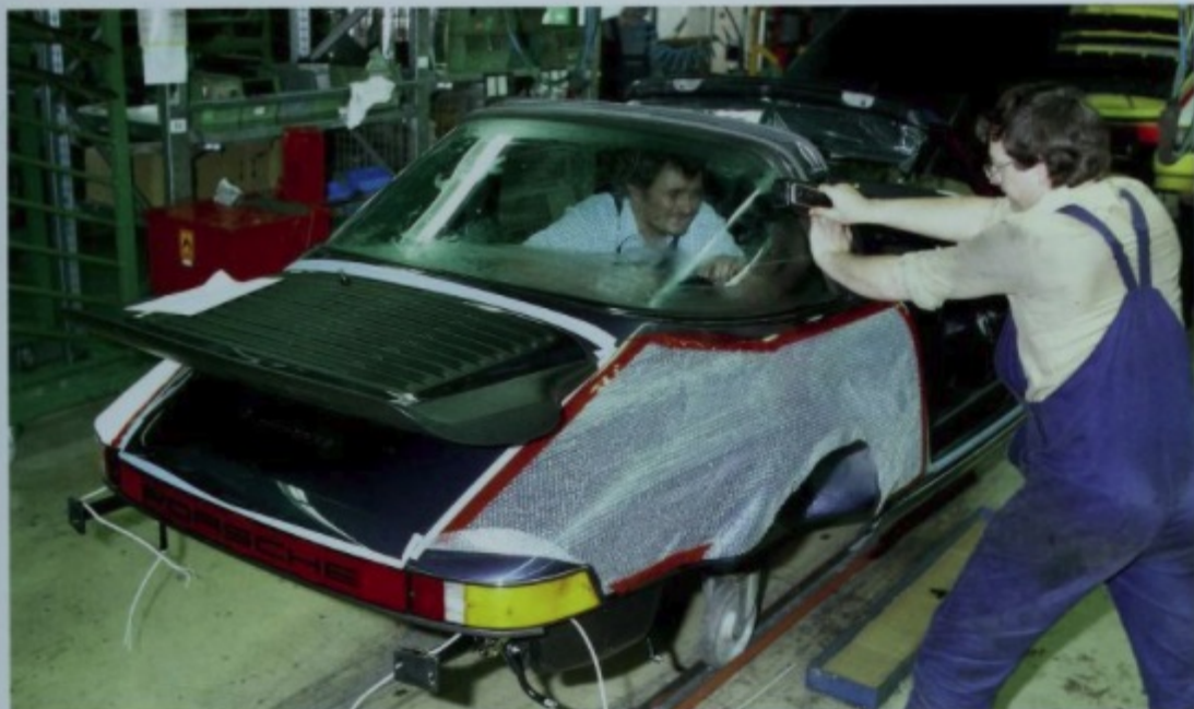
Grunt work. Installation of the rigid rear window requires a great deal of experience. Many a Targa backlight has been broken in the process.
