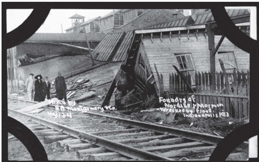
Foundry of Nordyke and Marmon wrecked by the 1913 flood (Indiana Historical Society, P0136).
