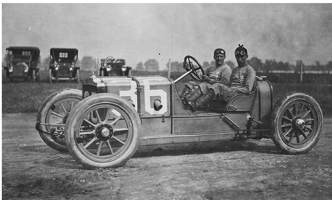
Fred Tone, driver and designer of the American Underslung cars, driving car number 36, a 50-horsepower American Underslung, at Brooklands in 1908 (with his mechanic).
