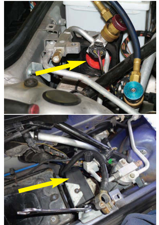
Two views of two different 996 alarm sirens (arrowed) show its mounting position on left-hand side of battery, and crammed in next to air-conditioning receiver-dryer
