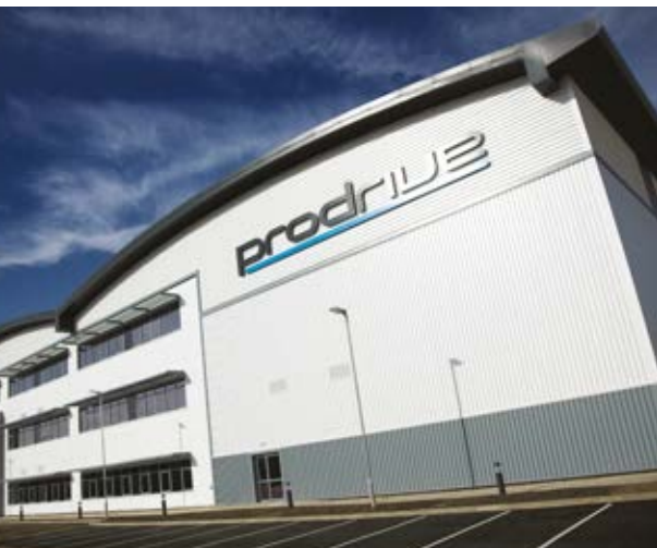
Prodrive was back in profit last year while the roof of its new headquarters in Banbury is now to be used to harvest solar power
