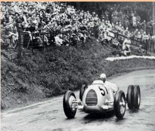
The Type C Auto Union used four rear wheels to help with traction in hillclimbs
