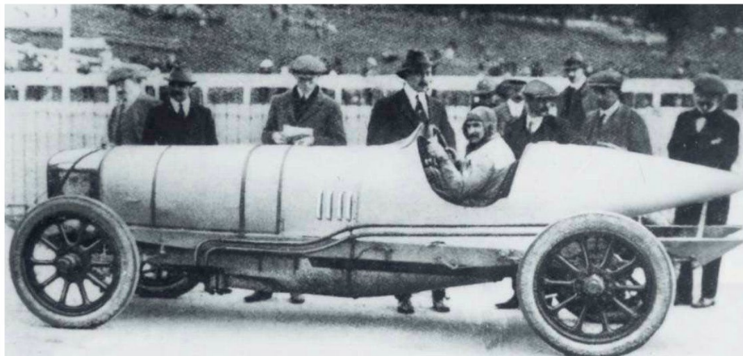
Jean Chassagne in the 9-litre V-12 Sunbeam which took the World One-Hour record at Brooklands in 1913. This was the first European V-12 engine.
