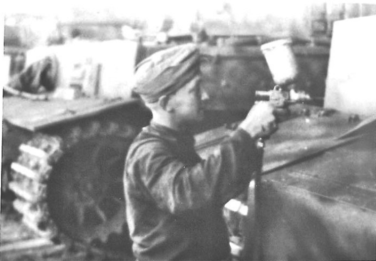
Units created their own camouflage patterns by spray painting Olivgruen (RAL 6003) and Rotbraun (RAL 8017) in irregular shapes onto the base coat of Dunkelgelb (RAL 7028) paint. (NA)
