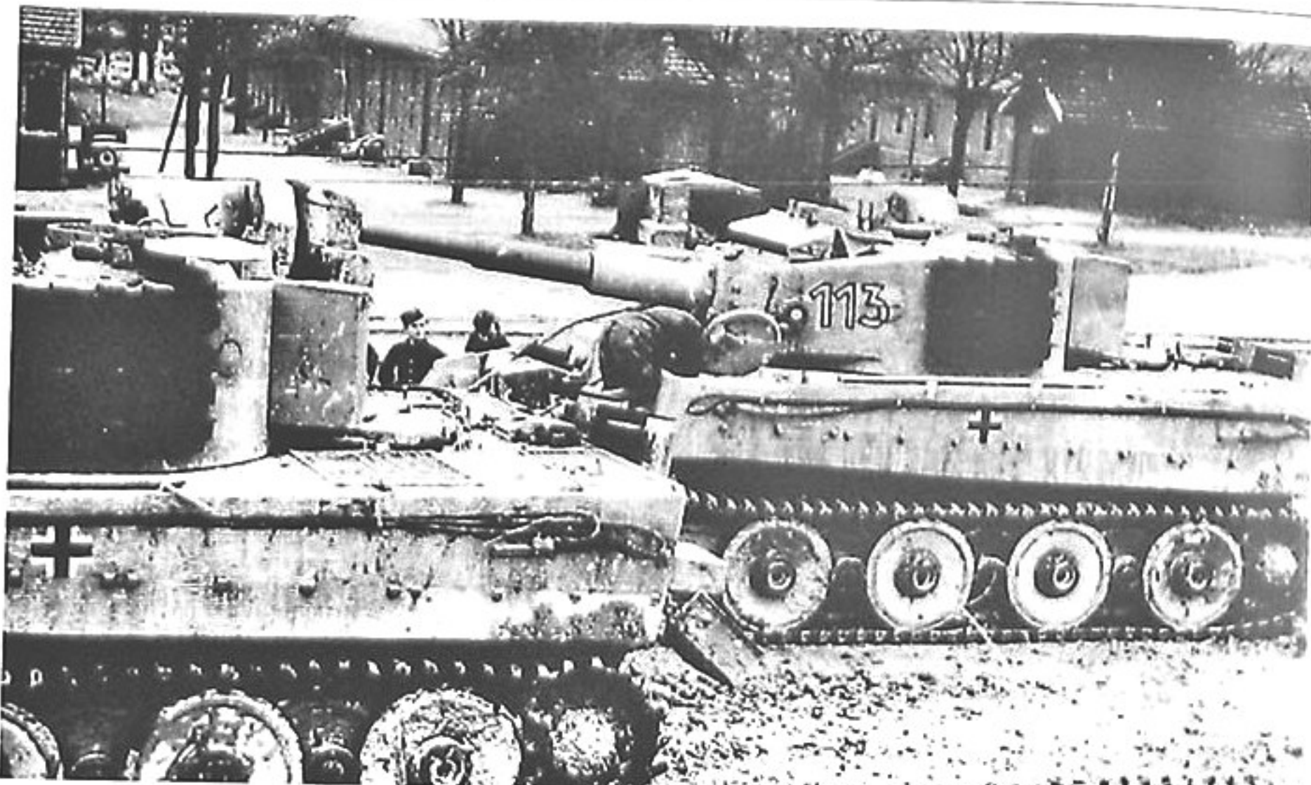
These two Tigers, completed in October 1943 and issued to s.Pz.Abt.501, still have fittings for Fefel air cleaners on the rear deck and pistol port plugs in the left turret side. (WS)
