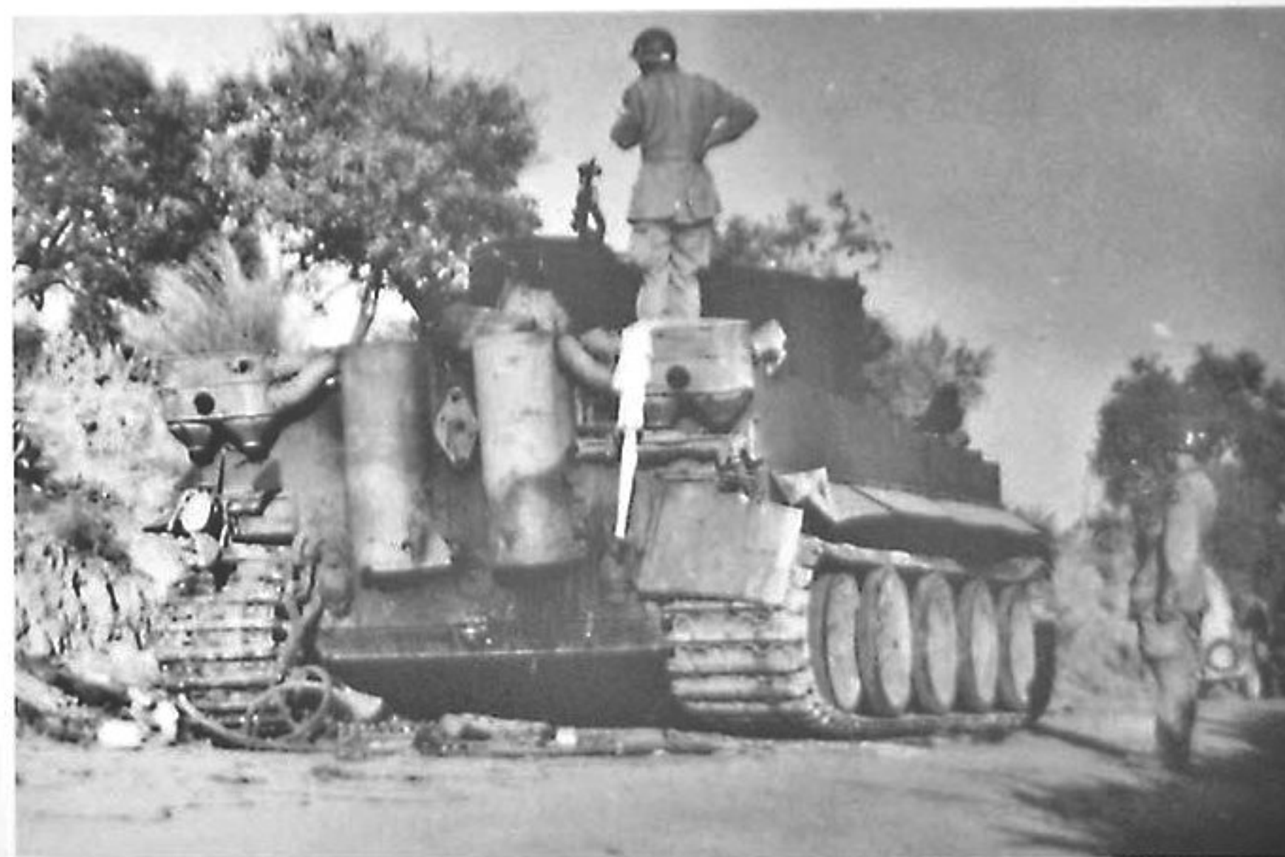
A Pz.Kpfw.Tiger Ausf.E (within Fgst.Nr. series 250200 to 250208 completed in April 1943 and issued to the 2.Kp./s.Pz.Abt.504 ) with three track holders on the right turret side and single upper chamber Feibel air cleaners. (NA)
