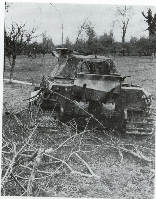
This rear view of a Tiger II fitted with a Porsche turret, shows the dual engine exhaust pipes located at the rear of the vehicle. Both the Tiger Is and early prototypes of the Tiger IIs had upright jacketed exhaust pipes. Field experience showed that hot exhaust gases were being sucked into the Tiger's cooling system causing numerous engine problems. To prevent this problem on the production models of the Tiger II, new unjacketed exhaust pipes—which were bent to direct the hot exhaust gases away from the vehicle's air cooling intakes—were fitted. The crew of the vehicle pictured have added what looks like a Tiger tank fender as an additional way of deflecting exhaust gases away from the engine cooling intakes. British Army Tank Museum
