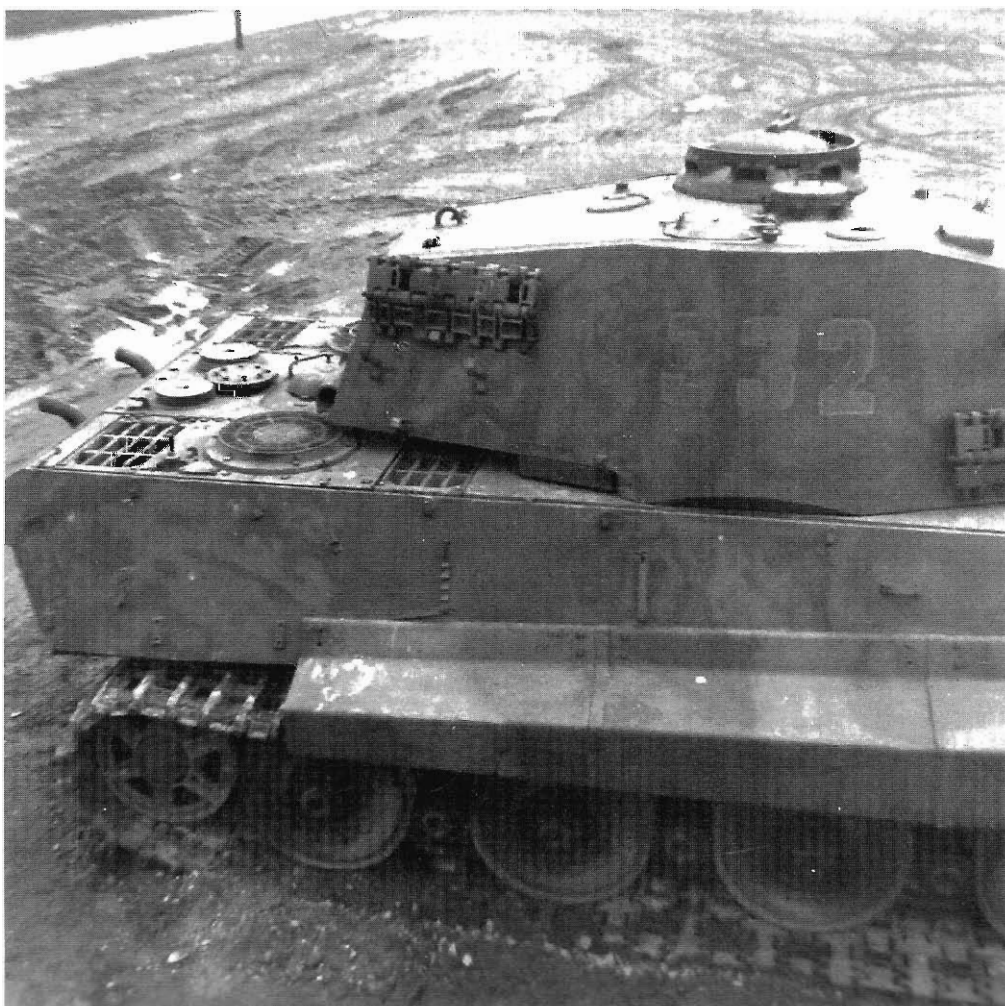
er Ausf.B (Fgst.Nr.280243, completed by Henschel on 11 September 1944) on display at the Aberdeen Proving Ground prior to cutting out the right side of the turret and superstructure for display inside the museum. It was completed directly after the order was issued to stop applying Dunkelgelb and did not receive a base coat of Dunkelgelb (RAL 7028) paint. An armor cap was bolted over the vent for the engine compartment on the rear deck. (APG)
