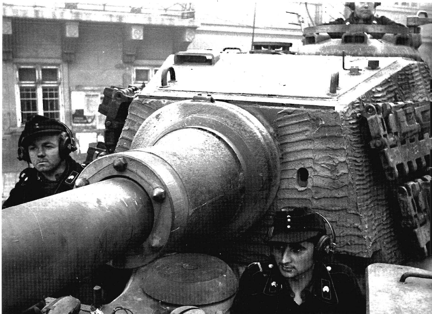
A closeup of the turret front of a Tiger Ausf.B , completed by Henschel in late August/early September 1944 and issued to the schwere Panzer Abteilung 503 . Apparently, the commander didn't like to fight buttoned up, as the hatch lid for the commander's cupola has been removed from the pivoting arm. (BA)
