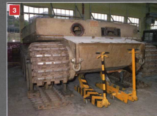
3 The hull is taken away to an empty vehicle workshop on the Bovington site to be worked on.
