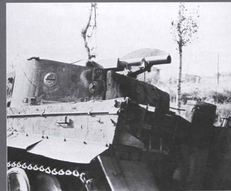
TOP The geared winding mechanism on the back of the Tiger's turret. The device was almost certainly manually operated.
