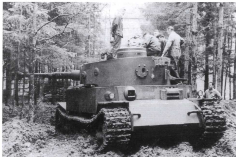
ABOVE In this photograph the Porsche design is fitted with the Krupp turret.
