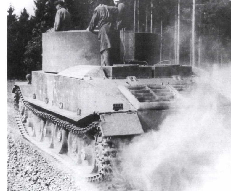
ABOVE VK 45.01 (P) – the Porsche design on trials, fitted with a dummy turret.
