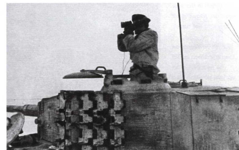
LEFT A Tiger commander looks out through the vision blocks in his cupola, binoculars to hand. He wears headphones and a throat microphone. As a system it had the advantage when in use of not transmitting background noise.
