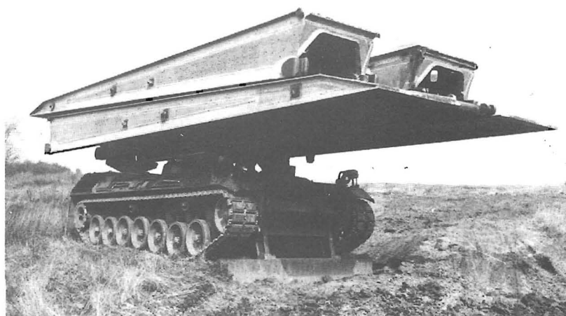
Right: Biber about to launch its bridge with the dozer blade being used as a brace.
