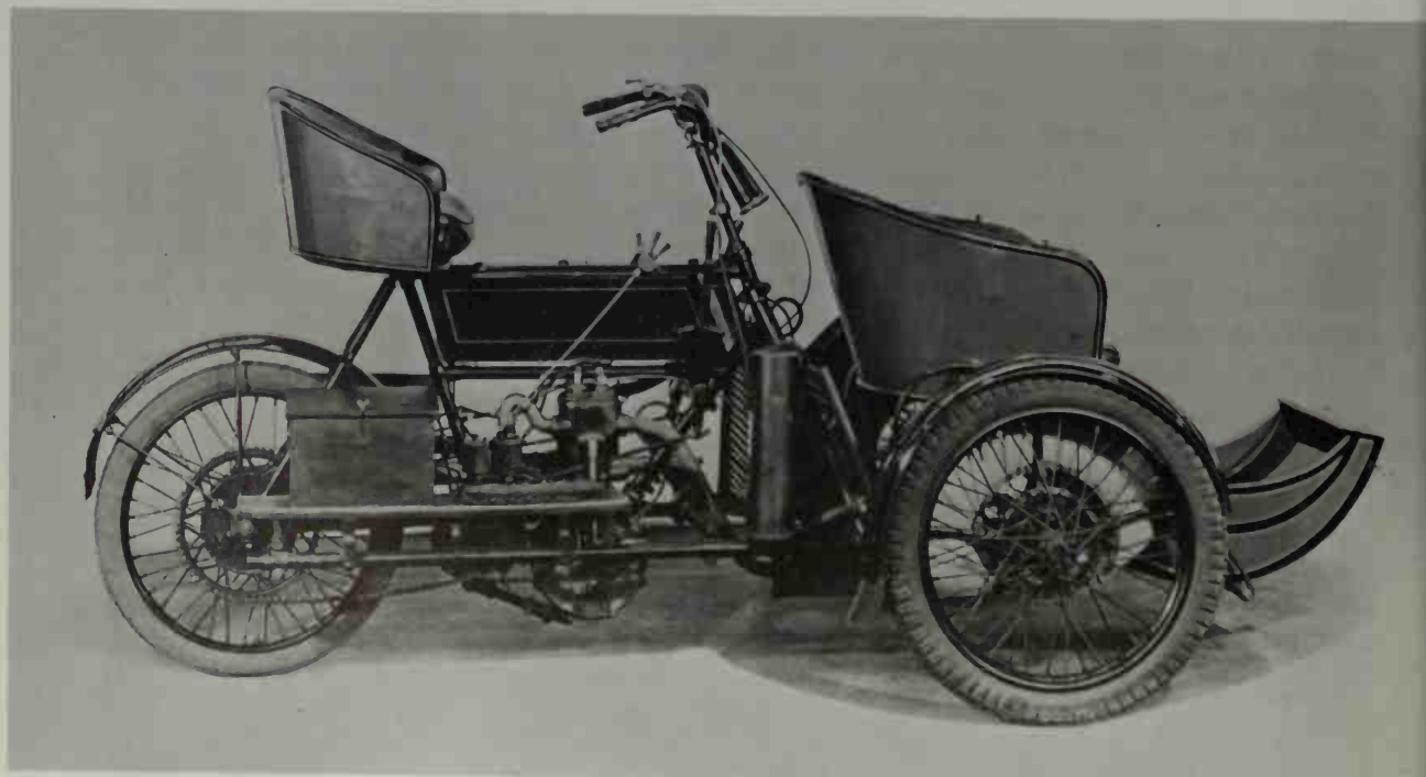
The 1904 Riley "Tricar" was obviously a bit behind the times although the single 4.5-HP cylinder
