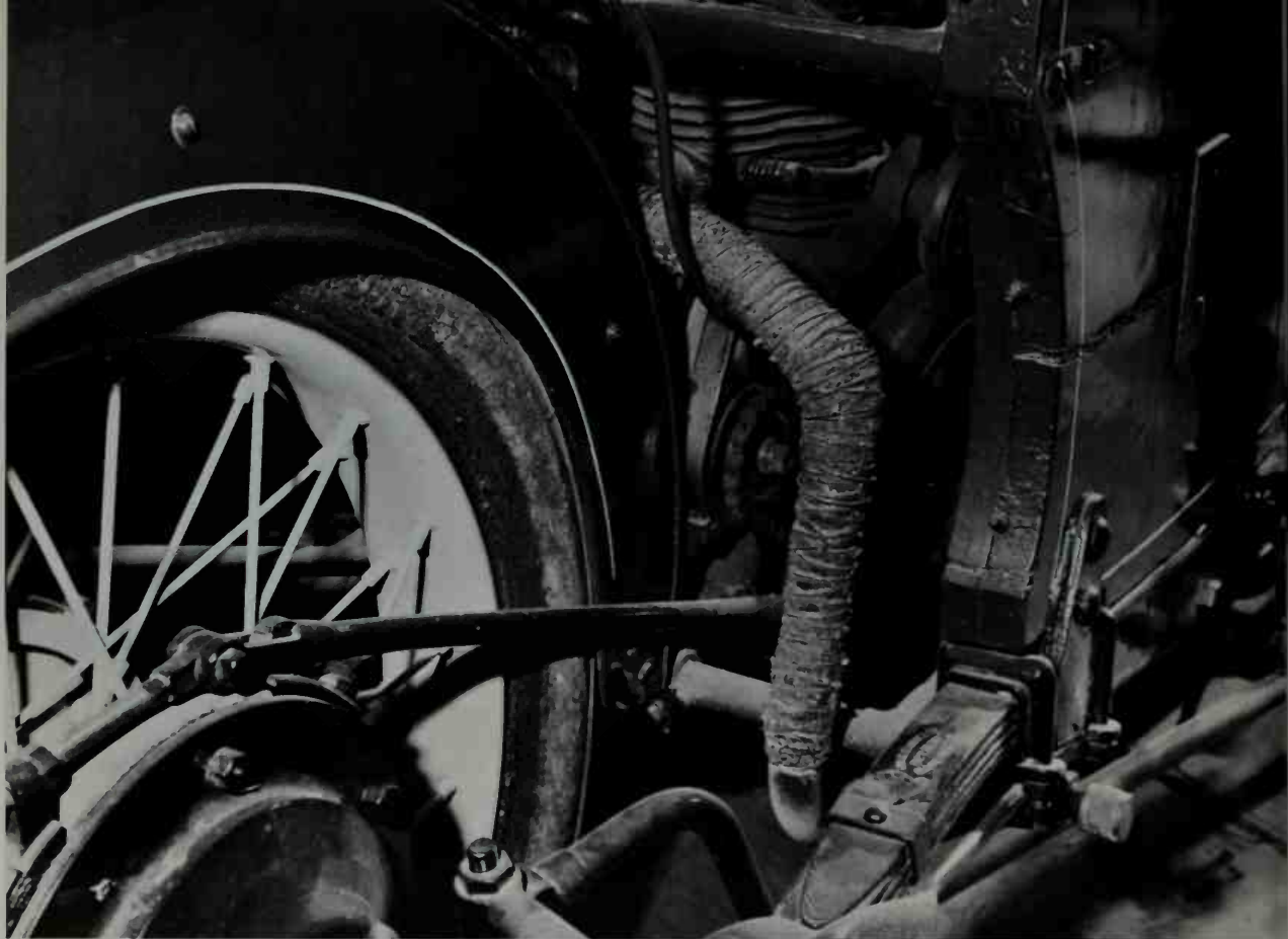
The 5-HP motorcycle engine and drive mechanism of the 1905 A. C. "Mighty Atom," the commercial forerunner of the first A. C. passenger carriage of 1910. The horizontal rod by wheel is the
