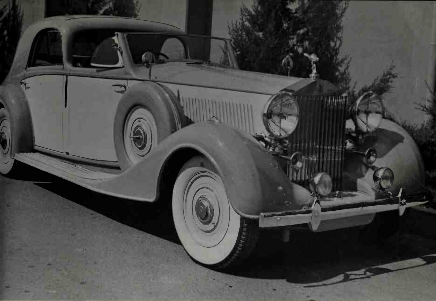
Rolls-Royce "Phantom III" Sedan de Ville with coachwork by Franay. Current during 1936-38, "Phantom III" had 7,340-cc., V-12 engines and
