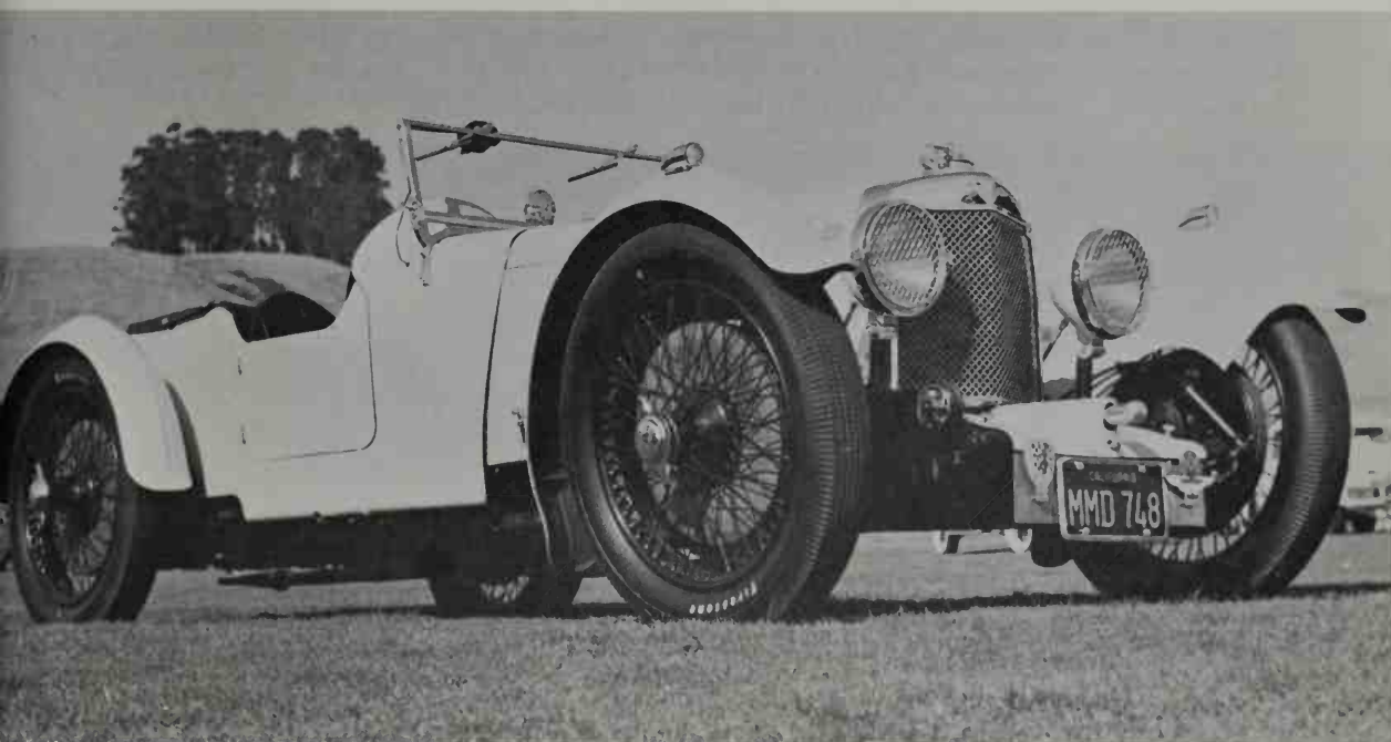
The 1.5-litre Aston-Martin "Le Mans" of 1932 had a 4-cylinder, single overhead-camshaft engine. One of these set a class speed record of 75.5 mph
