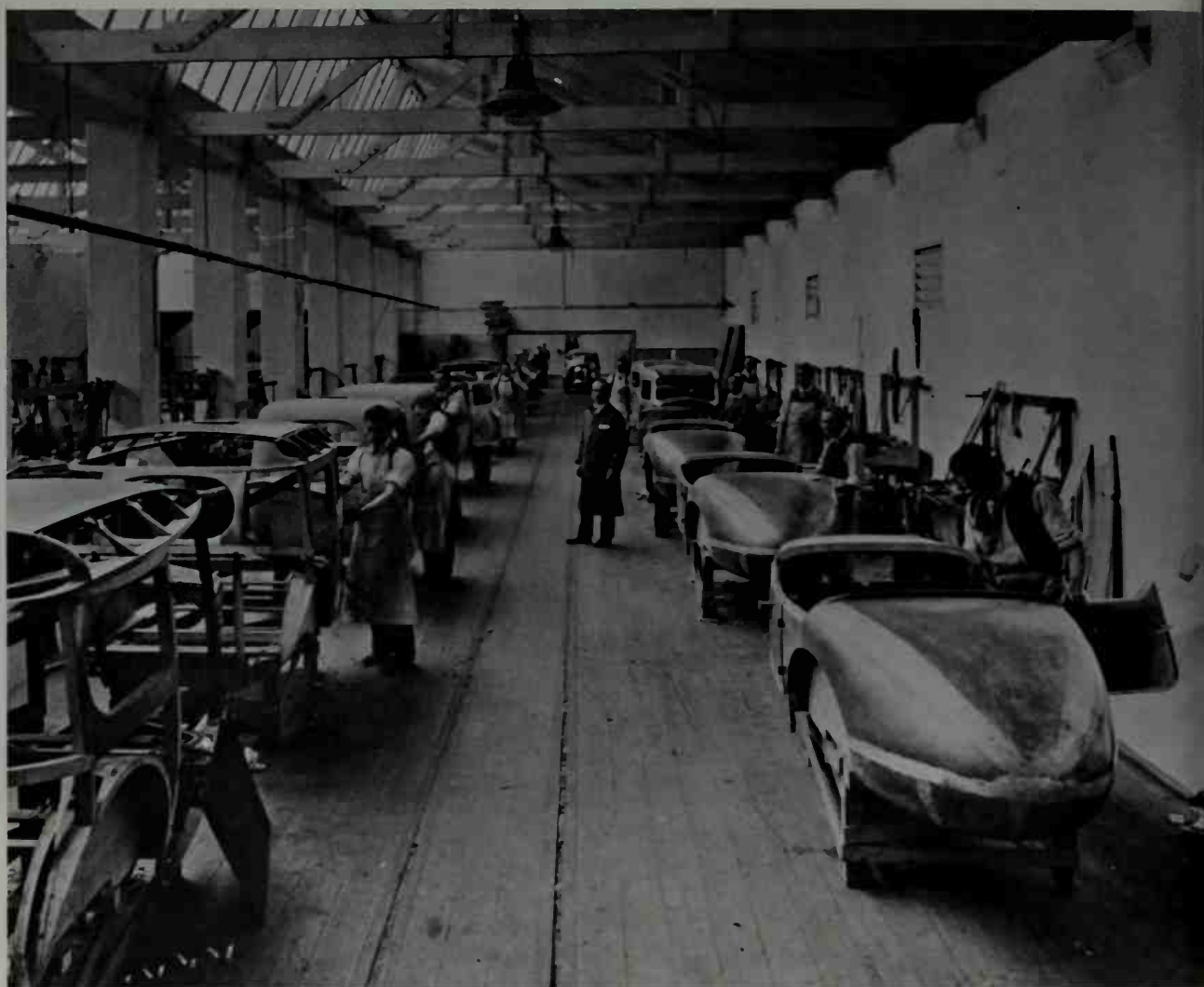
Basis of the future Jaguar cars was the Swallow coachworks. This 1929-30 photo shows wood-framed saloon bodies for the Austin "Seven"
