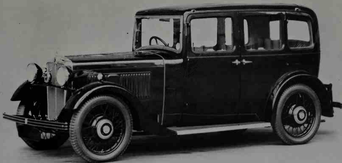
The 2,468-cc. Morris "Six" of 1933, a refined 6-cylinder (69 x 110 mm.) family car on a 118-inch wheelbase. Priced at about 350 Pounds up,
