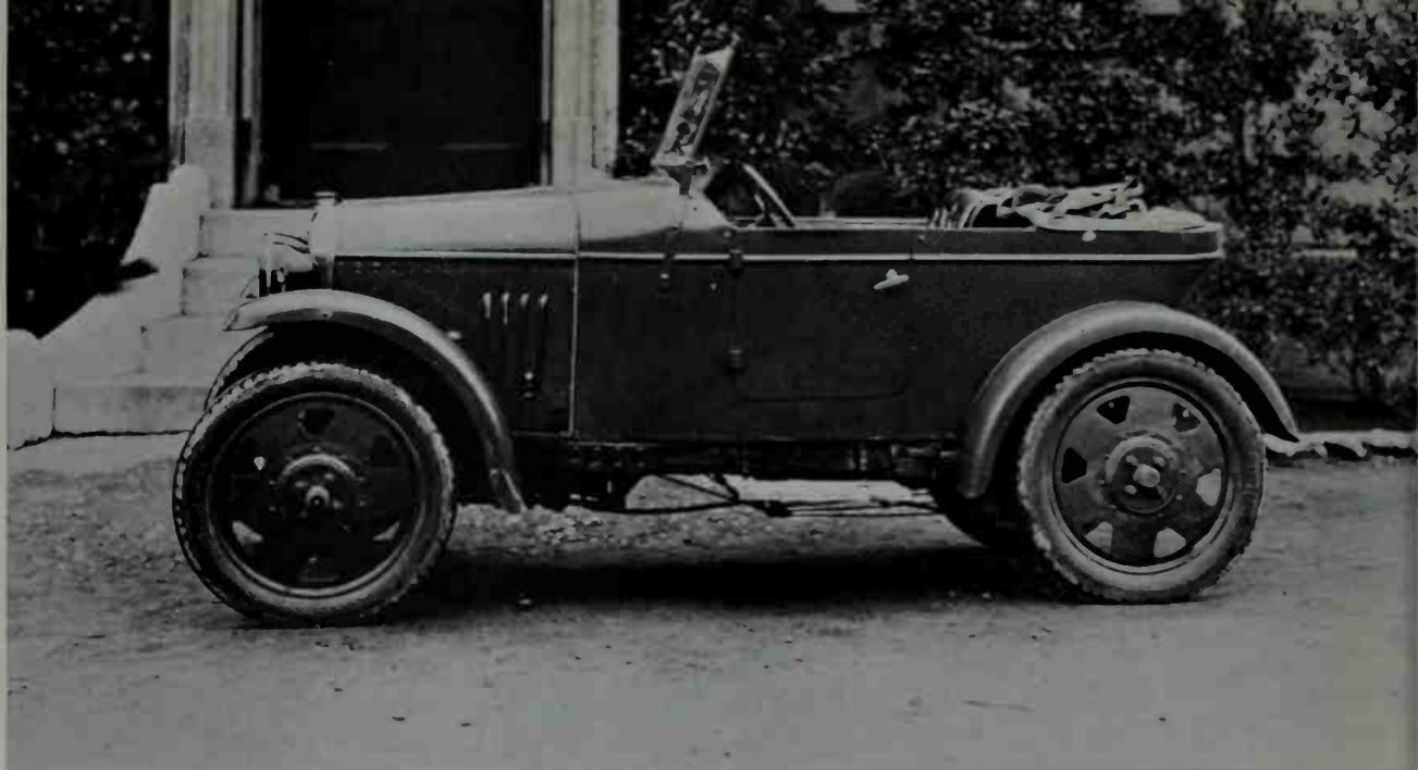
The "first trial model Datsun" was this two-seater of 1917. Note the loose brake cables beneath the stubby body. ( Jidosha Kogyo-Kia )
