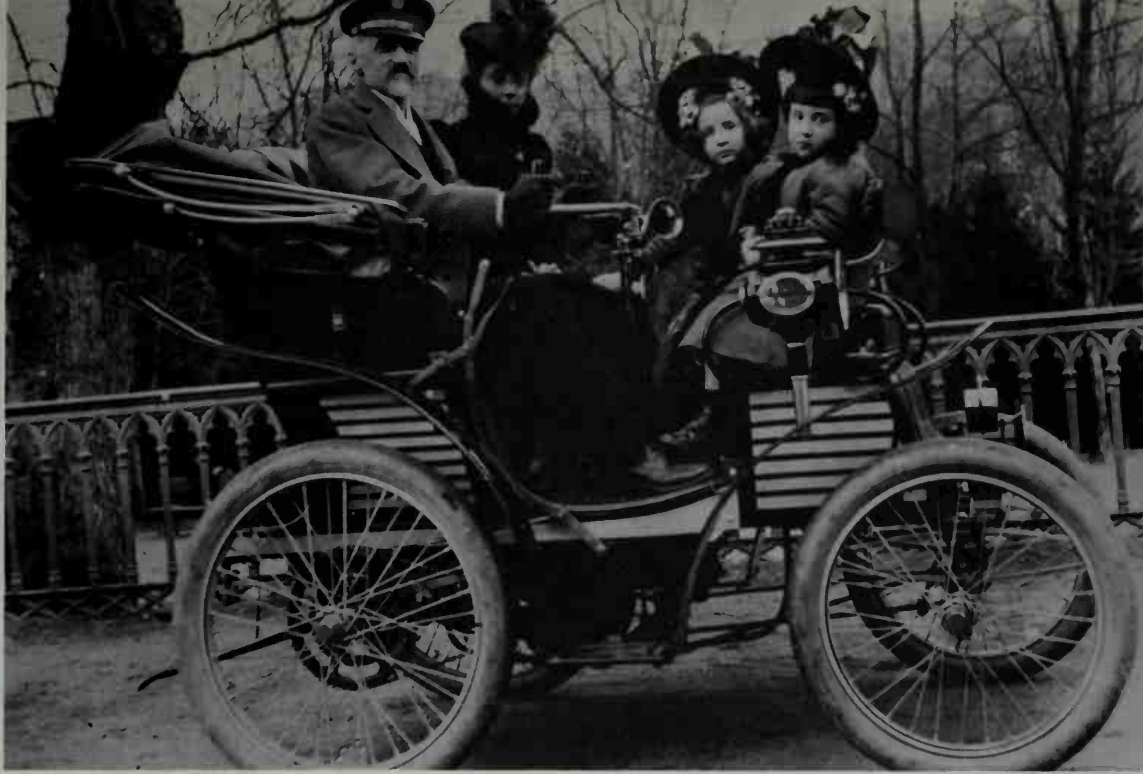
Ancestor of all modern Fiats were the high-riding 1899-1900 carriages powered by 679-cc., 2-cylinder, 3.5-HP engines. (S. A. Fiat)
