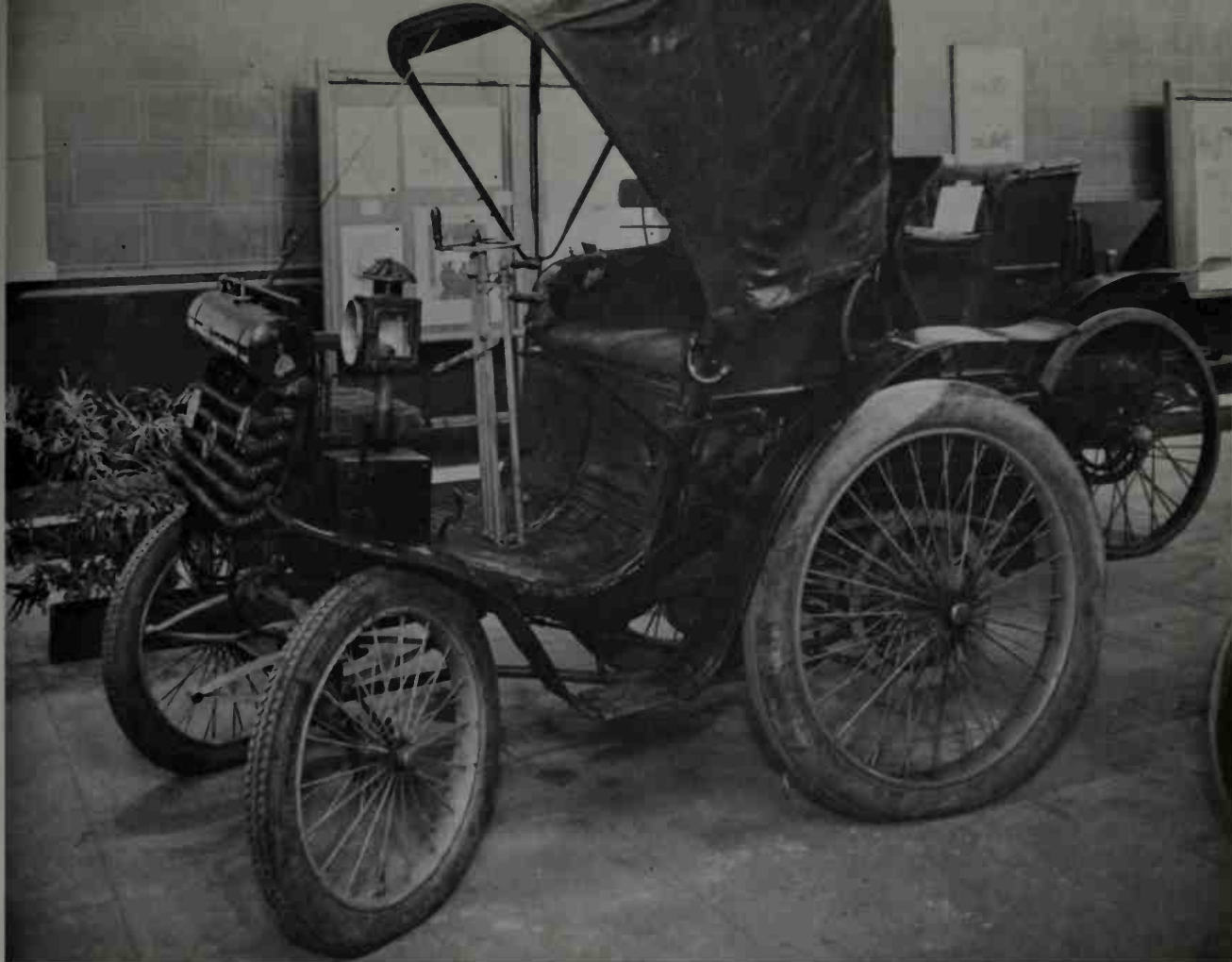
A 2¼ horsepower Daimler engine was used in this 1893 Peugeot. (French Embassy Press & Information Division)
