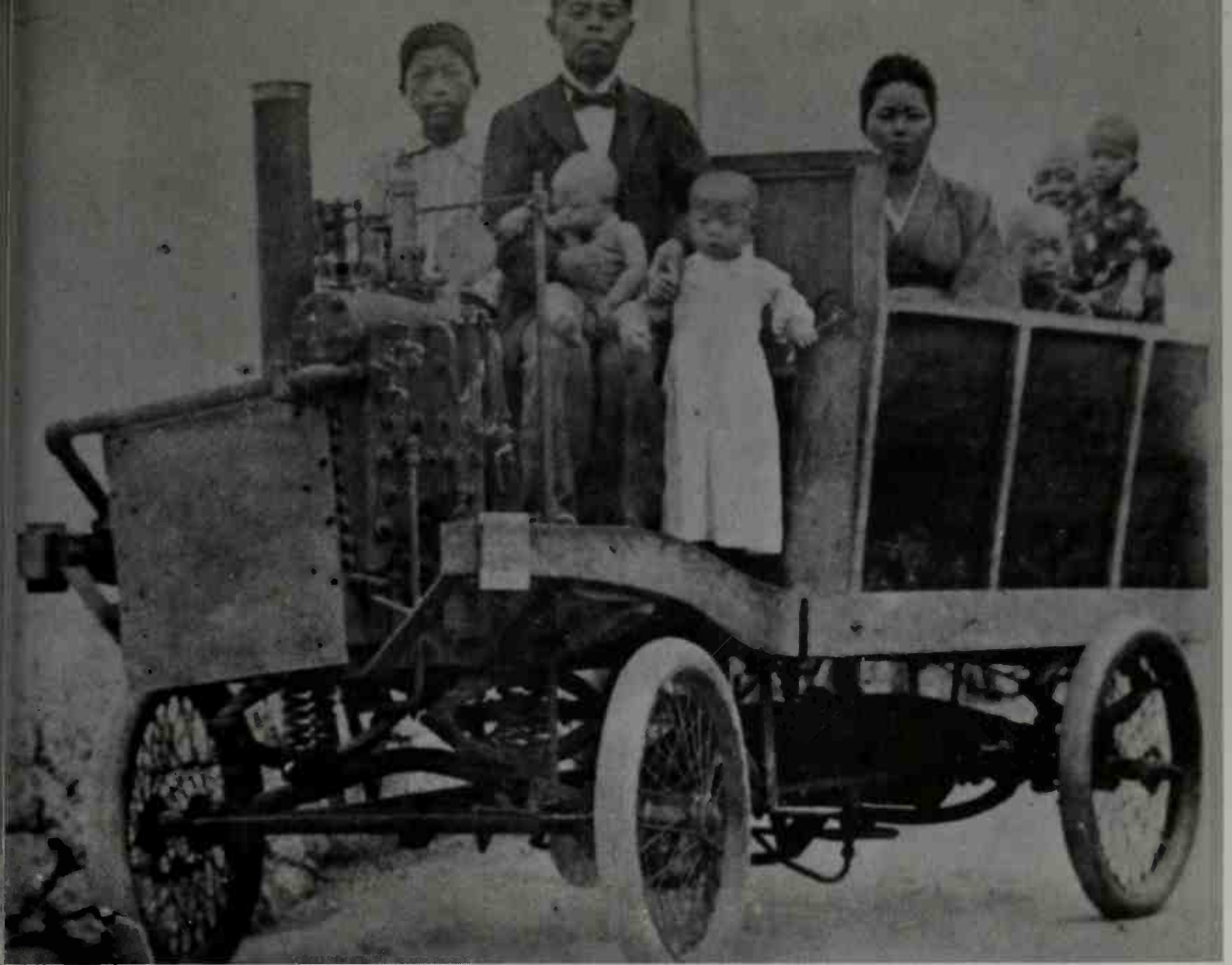
One of the first Japanese automobiles—possibly the very first—was this large 10-passenger steam car built by Torao Yamaba. The 2-cylinder engine
