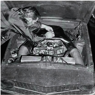
Ford supplied the Boss 302 race engines, but they were rebuilt by the teams. Here, a Bud Moore crew member secures the air cleaner assembly. Source Interlink Media Archives
