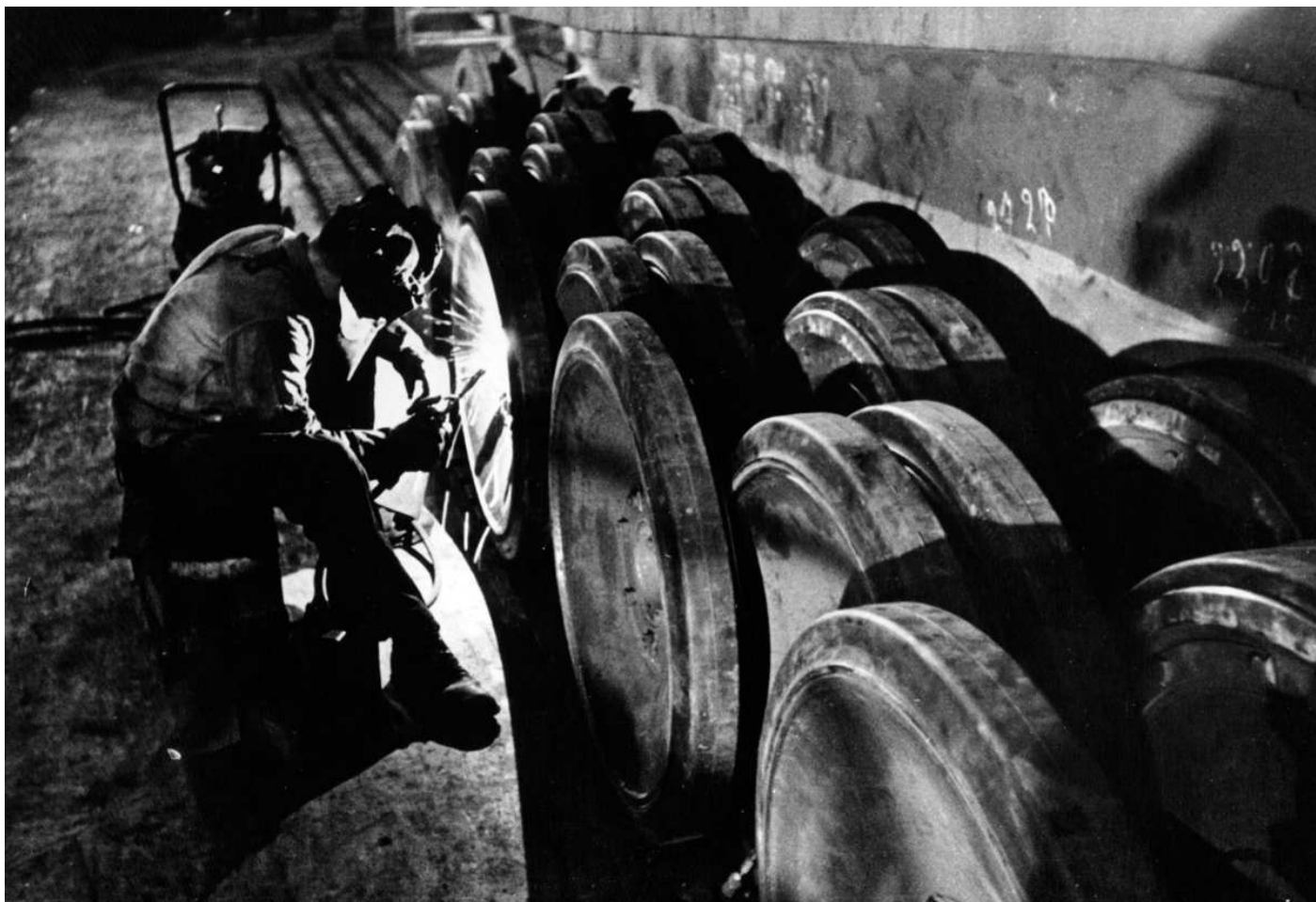
The interleaved running wheels before assembly. These provided stability and a smooth ride, but made maintenance difficult as all the outer wheels had to be taken off to access the inner ones and the torsion bars. (Panzerfoto)
