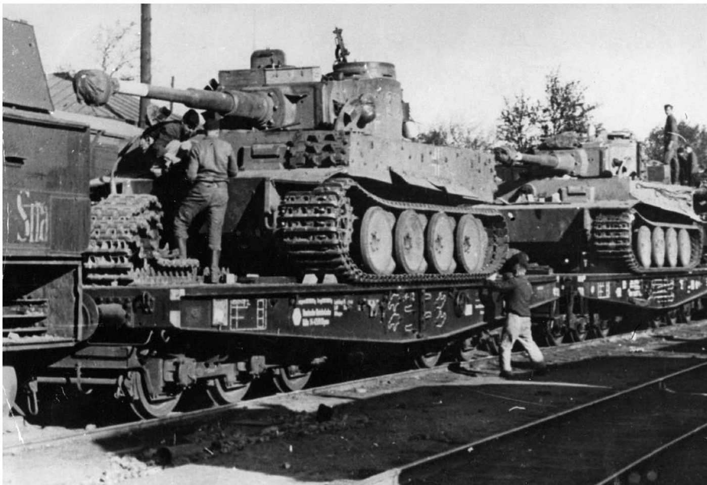
Tiger I tanks being transported on special railway lowloaders, October 1943. The wider combat tracks have been replaced with transport tracks. (Ullstein Bild via Getty Images)
