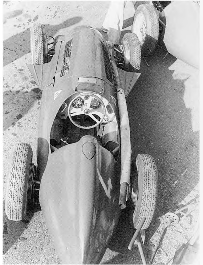
Overhead view of Fangio's car pre-practice. Even with the exhaust guard, it was still possible to get burnt on the right arm.
