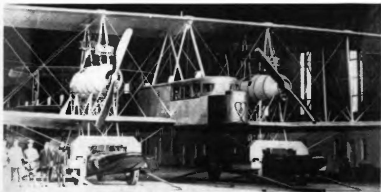
Germany's only successful giant bomber was the Zeppelin (Staaken) R.VI. Above is one of these machines mounted on two enormous floats, in which form it was known as the Type L. [H. J. Nowarra
