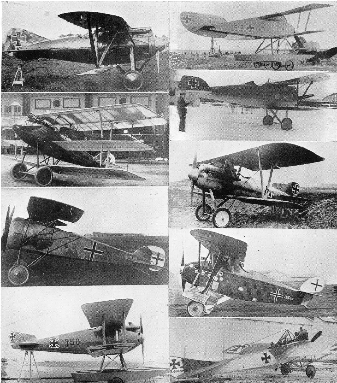
Top Left: Kondor D-7, 160 h.p. Mercedes, 1917. Next: L.F.G. Roland D-IV, 160 h.p. Mercedes, 1917. Next: L.F.G. Roland D-XVI, 160 h.p. Siemens or 170 h.p. Goebel, 1918. Bottom: L.F.G. Roland W.1, 160 h.p. Mercedes, 1917. Top Right: Luft Torpedo 5D1, 150 h.p. Benz, 1916-1917. Next: L.V.G. D-II, 160 h.p. Mercedes, 1916. Next: L.V.G. D-IV, 190 h.p. Benz, 1917. Next: L.V.G. D-VI, 190 h.p. Benz, 1918. Bottom: L.V.G. E-VI, 160 h.p. Mercedes, the first two-seater with both fixed and flexible guns, 1915.
