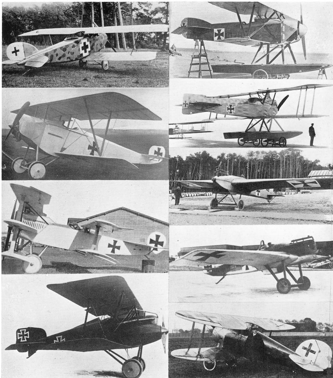
Top Left: Zeppelin Dornier CL-II, 240 h.p. Maybach, 1918. Next: Euler D-I, 100 h.p. Oberursel (a Nieuport copy), 1916. Next: Fokker V.8, 120 h.p. Mercedes, Experimental Quintuplane, 1917. Bottom: Friedrichshafen D-I, 160 h.p. Mercedes, 1917. Top Right: Hansa-Brandenburg W.16, 160 h.p. Oberursel, 1916. Next: Hansa-Brandenburg W.25, 150 h.p. Benz, 1917. Next: Junkers J-I 'Blechesel' (Tin Donkey), 120 h.p. Mercedes, 1915. Next: Junkers E-II, 160 h.p. Mercedes, 1916. Bottom: Kondor D-I, 110 h.p. Oberursel, 1917.
