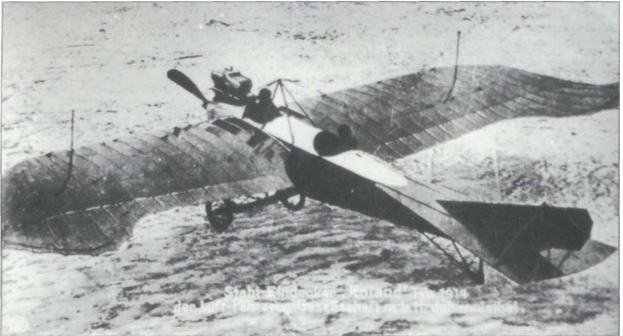
Above One of the so-called Steel Taubes , built by LFG Roland during 1914. Employing a steel tube structure in place of the Etrich's original wooden one, the 100hp Daimler having now become a 100hp Mercedes D I. Despite these changes, performance, or at least the 71 mph top level speed appears to have changed little. Note the retention of wing warping and the distance between pilot in the rear and the front seated observer, something that could not have helped in-flight communications. (Cowin Collection)
