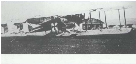
Although always overshadowed in the public eye by the Gotha name, the Friedrichshafen G III equipped three of the eight German bomber wings at the time of the Armistice. Larger and heavier than the contemporary Gotha G IV, the G III carried a far heavier bomb load and seemed far less susceptible to the landing gear failures that constantly beset the Gothas. With a 3-man crew, the G III was powered by two 260hp Mercedes D IVs and could carry up to 3,300 lb of bombs. Armed with two or three 7.92mm Parabellums, the G III had a top level speed of 87mph at 3,280 feet, along with a duration of 5 hours, implying a tactical radius of action, with full bomb load, of around 140 to 145 miles. Deployed initially in mid-1917, the G III and G IIIa went on to equip KG 1, KG 2 and KG 4 during 1917 and 1918. (Cowin Collection)
