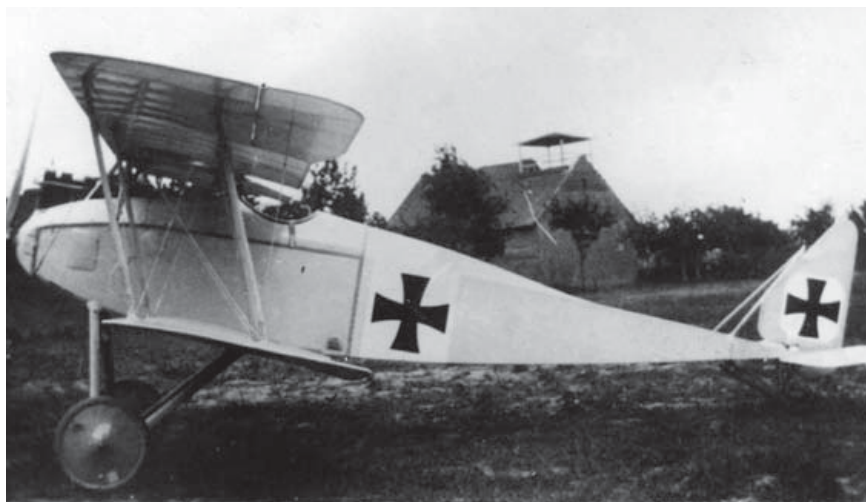
The single-gunned Halberstadt D.II was at the forefront of Germany's focus on in-line engine, biplane fighters. Although its performance was praised beyond that of the Fokker Eindecker , there remained calls for airplanes with increased engine power and a second machine gun.
