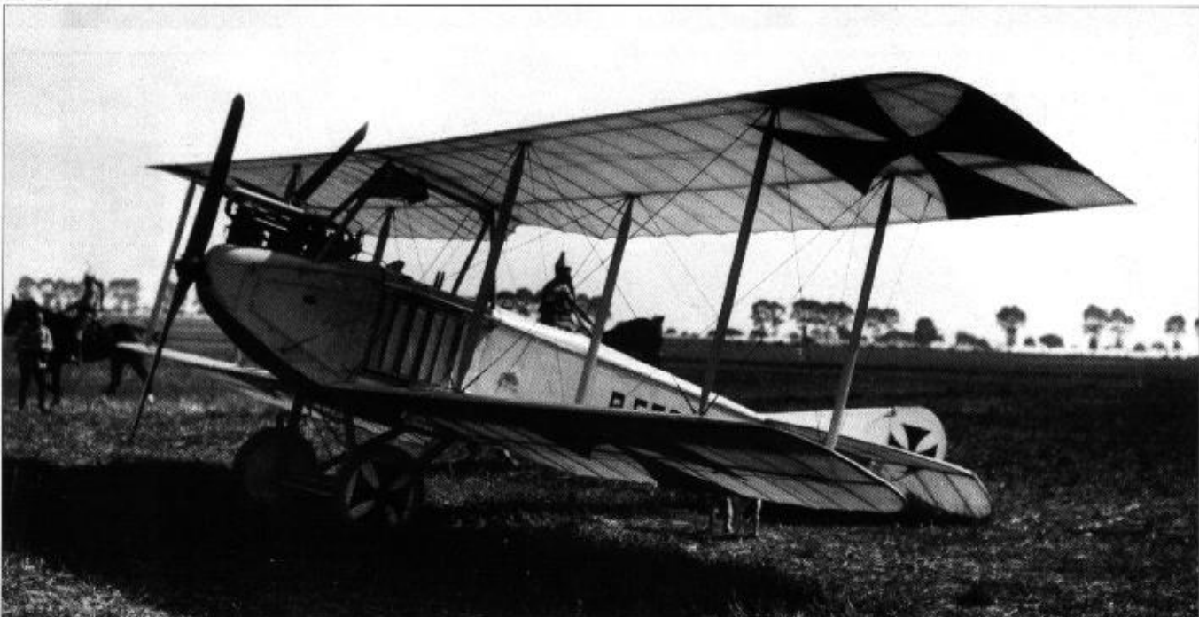
Page 26: 52). Aviatik B.576/15 (P 15) in a common predicament. This version does not have a gravity tank or button rudder.
