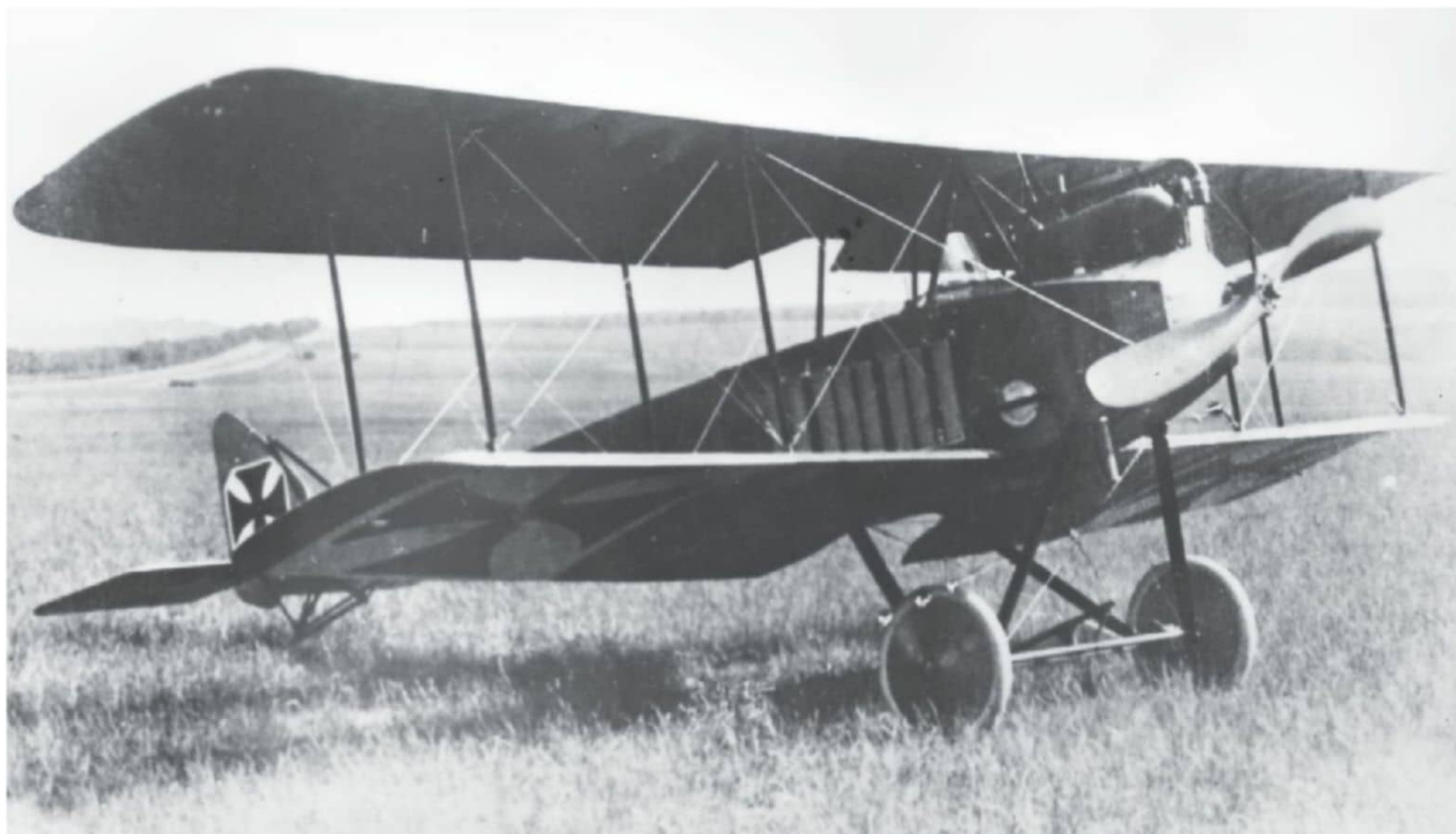
Above: The first Halberstadt D.I prototype was a downsized version of the B.II, reputedly built towards the end of 1915 suggesting that Halberstadt were the first German company to develop a scout in a biplane configuration
