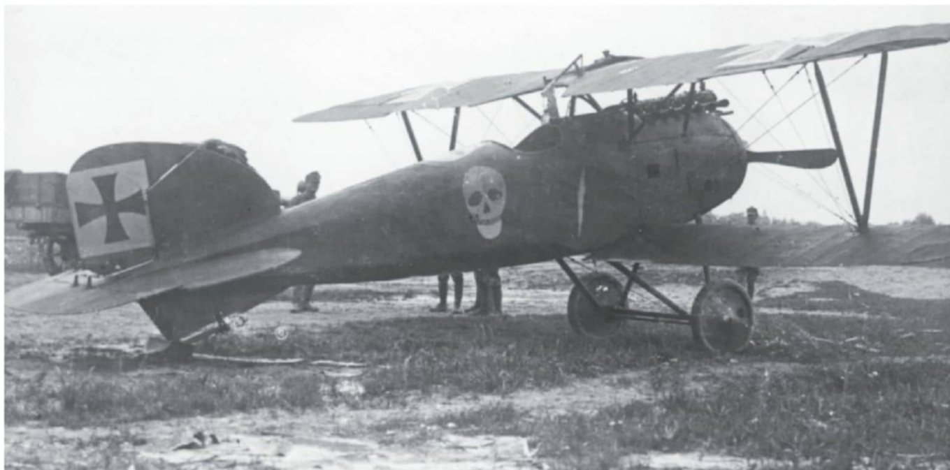
Above: A well-known photograph of Godwin Bromowski's last Albatros at Portbuffole in June 1918. D.III (OEF) 153.209 was over painted red with Bromowski's customary death's head shroud visible on the fuselage. Note the Aldis telescopic sight taken from a British aircraft and mounted in front of the cockpit. The device mounted on the upper wing is probably a flare pistol
