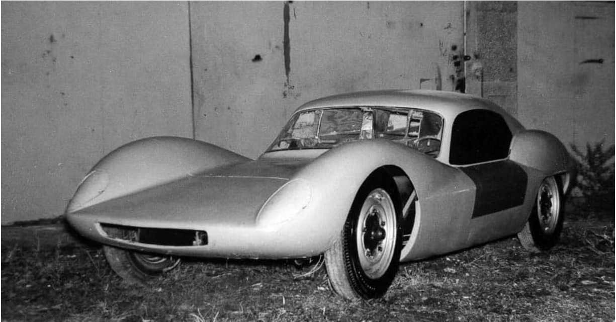
1966: the Mk II Sabel, a coupé of which John says he built just the one. It was built on a modified VW Beetle floorpan able to use VW, Porsche or Corvair power. (Sab)
