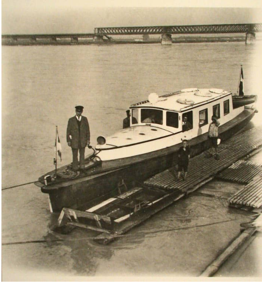
1920 on the Danube: motor yacht 'Argonaut' with a 220hp Austro-Daimler six-cylinder boat engine; aboard the boat is owner Ing Theo Weichmann. The engine and boat bodies of the motor yacht 'Argonaut' were built under the direction of Ferdinand Porsche in Wiener Neustadt near Austro-Daimler and the OEFFAG (Austrian Airplane Factory). The 'Argonaut' had berths for four persons. Length: 14.81m; weight: 6500kg; engine power: 220hp at 900rpm; speed: 22 knots (40.7km/h); action radius: 500 nautical miles. (P)
