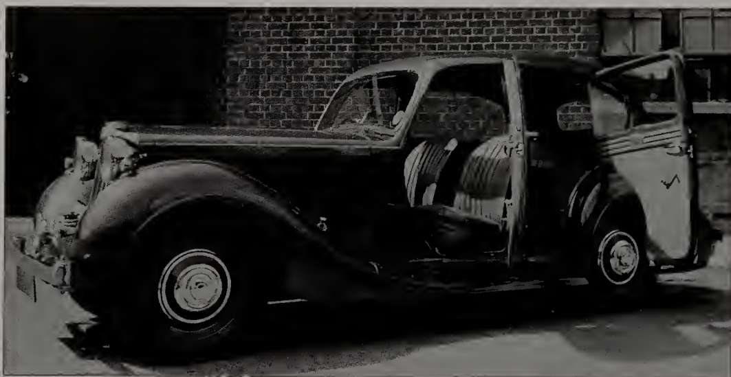
The 2-Litre, powered by the 56bhp sidevalve engine from the Humber Hawk.
