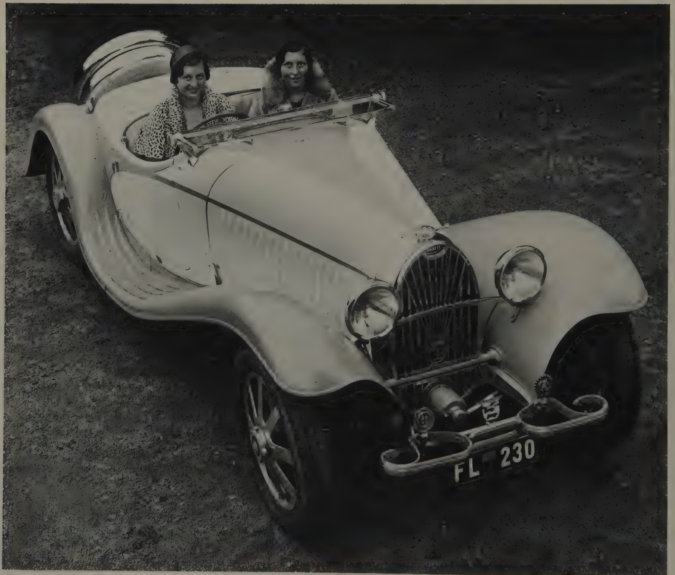
The sloping cowl in front of the radiator made the four-wheel-drive 53 different from other racing Bugattis. The Type 55 below although more flamboyant has much the same lines as Jean Bugatti's doorless two-seater.
