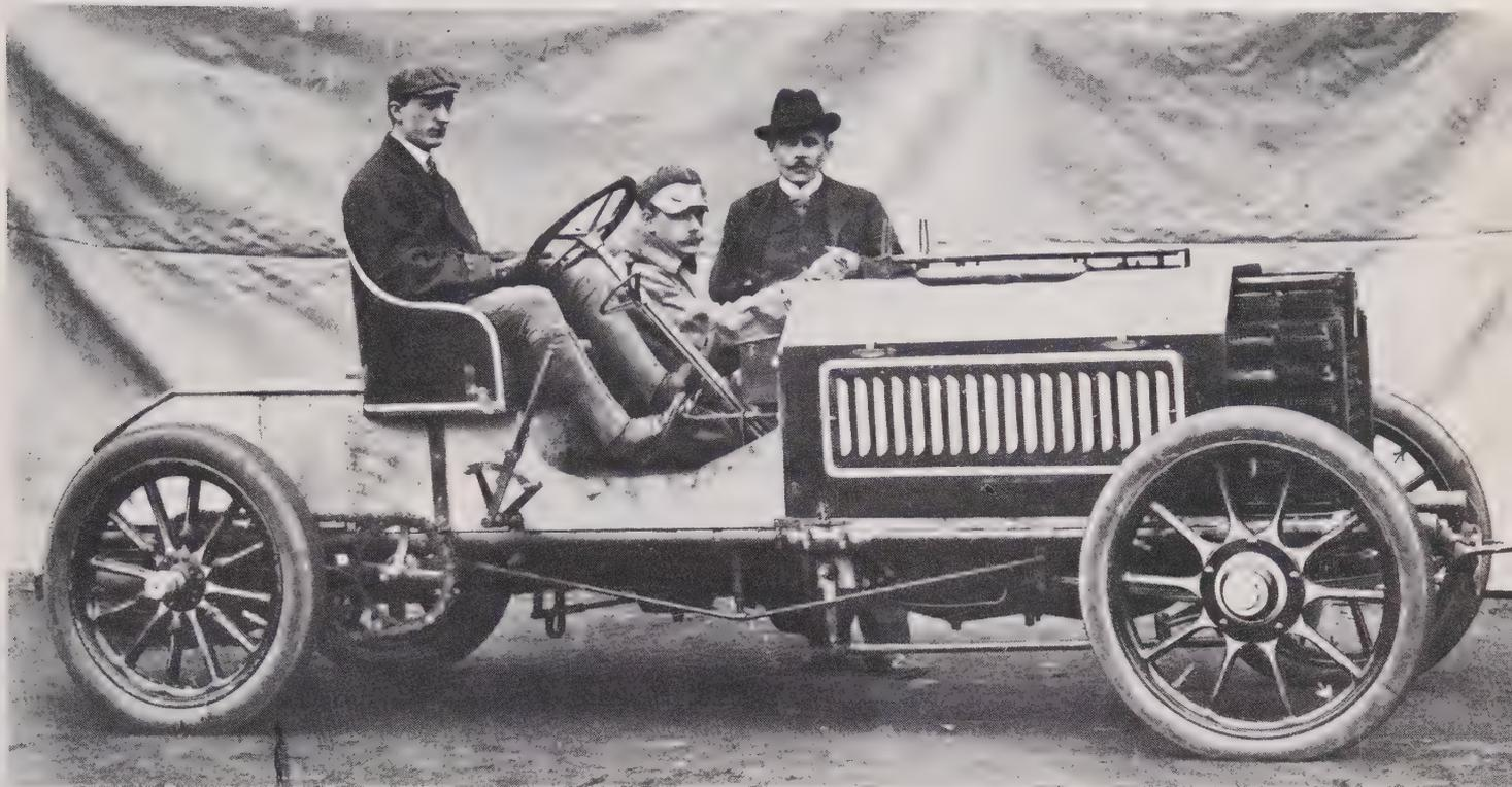
*Type 5 Paris–Madrid car. This is in the modified form with the driver placed normally, after the authorities would not let Bugatti drive the car in the original position at the rear, as used in the smaller racing car. The car had a tubular frame and an engine of 160 × 160 mm (12.86 litres). What became of it is not known.*
