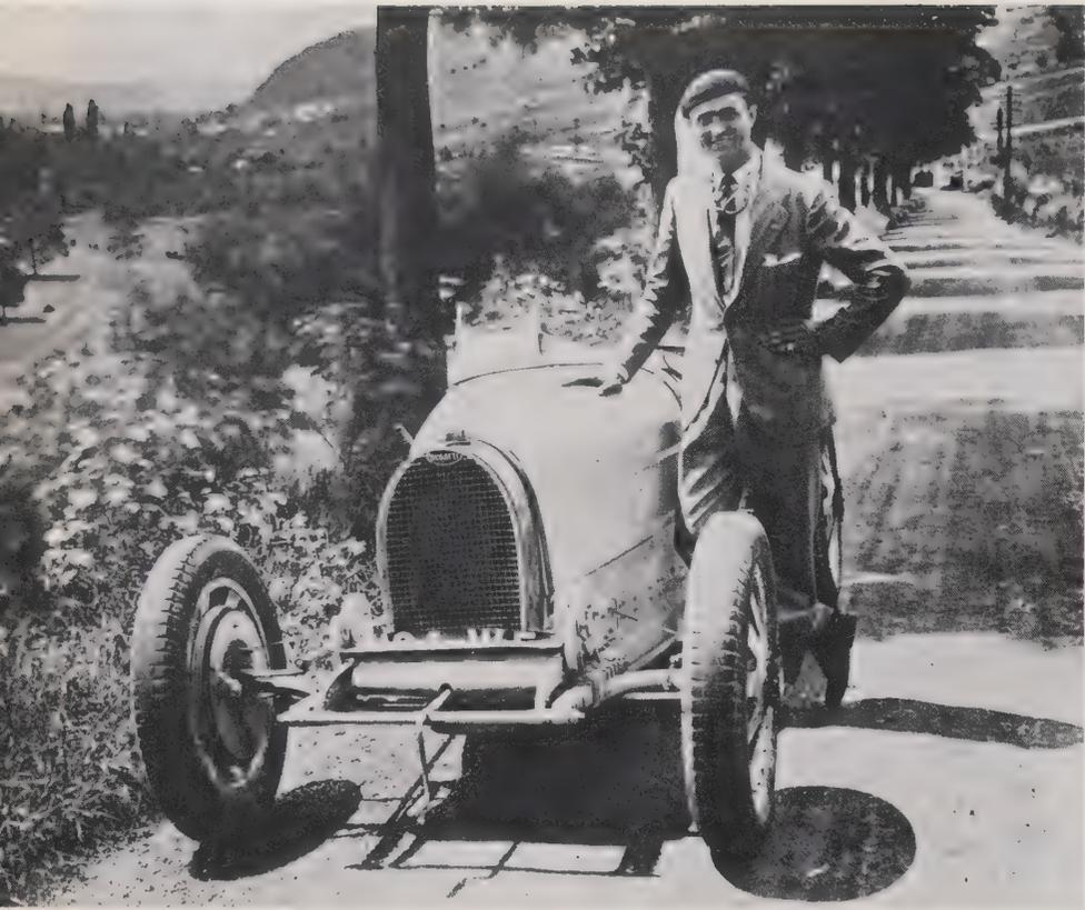
*Chiron at Molsheim testing the first T35B 2.3 litre supercharged model, now with big brakes.*
