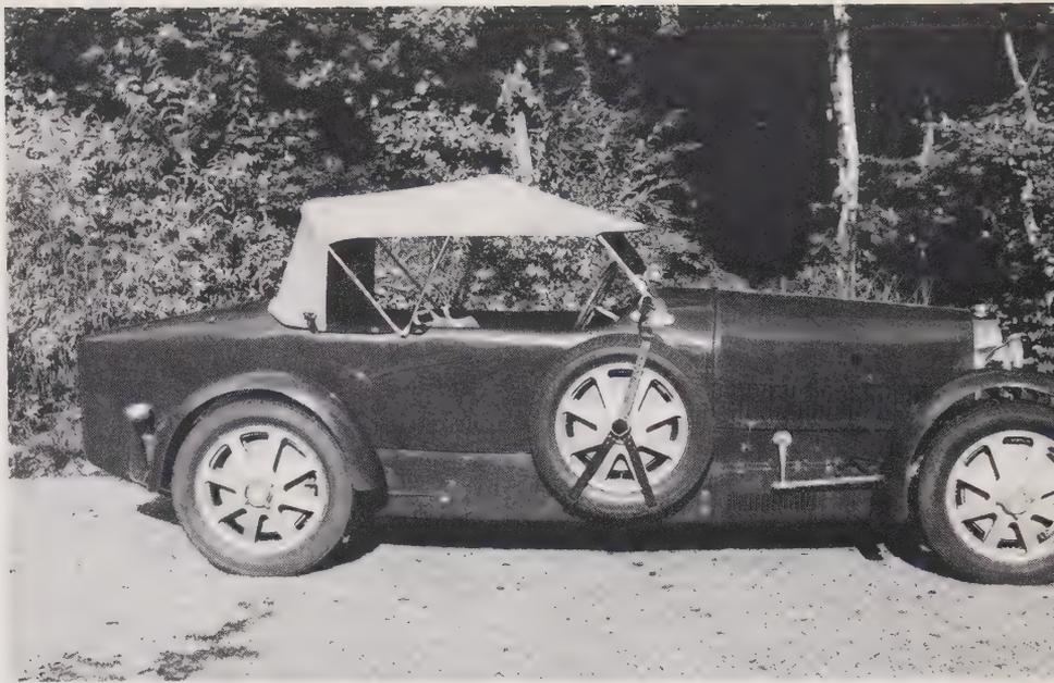
*The standard body has a fixed windscreen, and wipers were not fitted. The single door contributes to body stiffness.*
