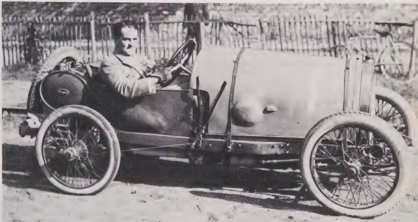
*What is now commonly called a Brescia started as a Type 13 with bolster tank at the rear and the minimum of bodywork, and, in its 1920 Le Mans form, is strictly a '16-valve'. Here is Pierre de Viscaya before the race. The engine was 66 × 100 mm for this race, but was soon enlarged. The first models had a single magneto, but later for the 1921 race at Brescia, where it swept all before it, it had twin magnetos mounted in the dash, and a ball bearing crankshaft.*
