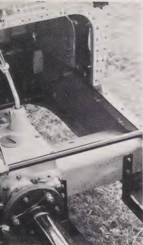
*The gearbox straddled the frame, and was bolted to the webs perhaps to stiffen the frame a little. The gear lever had a ball-end.*
