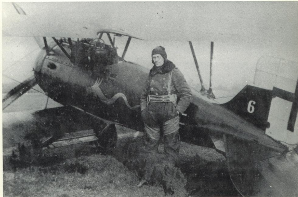
104. This squat little aeroplane is one of the early prototypes of the Siemens Schuckert DIII and DIV aircraft, which many air historians consider to have been the best German fighters to reach operational status. For some reason, the aircraft continued to be manufactured until the summer of 1919, and at least one DIV survived until 1926 in Germany. (Paul Leaman)
