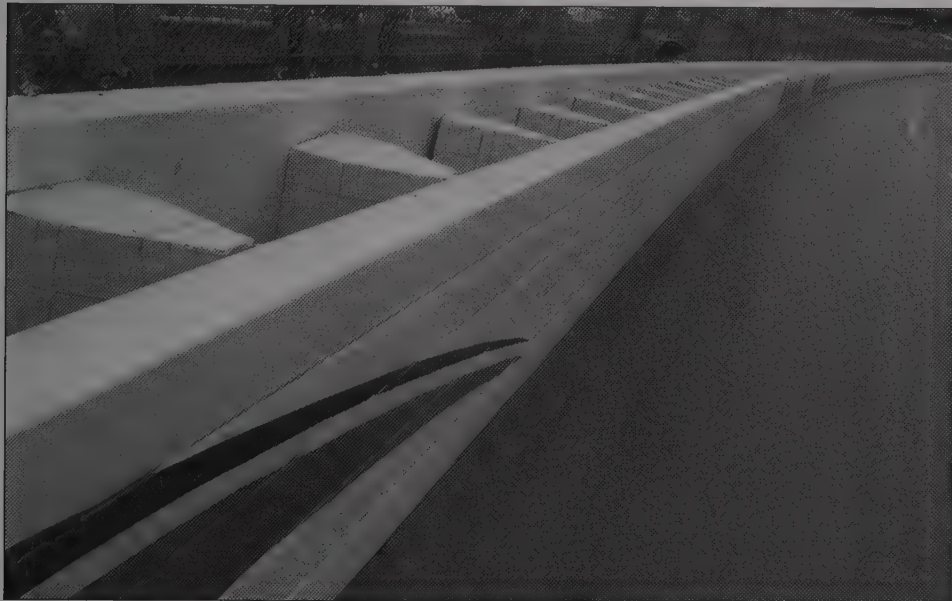
The MwRSF broke new ground in 1998 in an effort to improve driver safety. The MwRSF was selected by the IndyCar Series, the Indianapolis Motor Speedway, and NASCAR to develop, test, and evaluate safety features for high-speed race tracks. It developed the SAFER barrier for use on high-speed oval race tracks. (Courtesy of Brian Cantoni.)
