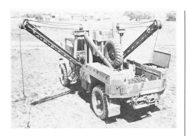
This shot of a CMP Chevrolet C60S 3 ton breakdown truck clearly shows the layout of the Holmes swinging booms and equipment lockers.
