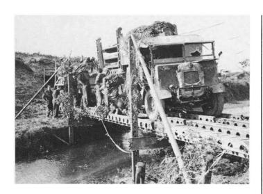
An Albion BY5 with folding bridge equipment body in difficulties crossing the river Garagliano in Italy. A Diamond 'T' 6 ton wrecker has come to the rescue.
