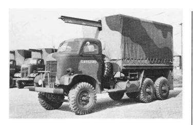
The Dodge WK-60 3 ton  $6 \times 4$  breakdown, built to British requirements to supplement UK production. It incorporated right-hand drive and the rear bogie was driven via a Thornton power divider. British-built body was fitted to chassis in the UK.
