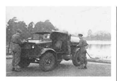
An MW 200 g water tanker of the Aldershot District filling from a local pond. Samples are lined up on the bonnet to undergo purity checks.
