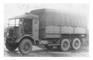
A late production Albion BY5  $6 \times 4$  3 ton with the all-steel GS body which superseded the wood body in 1944. A hip ring has also been fitted to the cab tilt.
