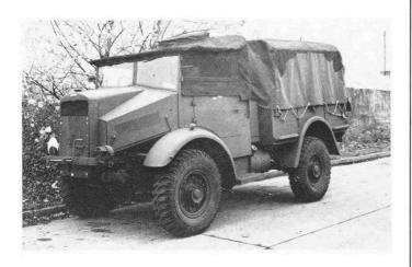
The Morris-Commercial C8|GS 15 cwt 4 × 4 was introduced in late 1944. It could be fitted with either wood or steel GS or light warning radar body. It was noisy, slow and vibrated terribly, at least the one the author drove did.
