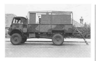
A standard Bedford QLC with mobile kitchen equipment installed. These vehicles provided cooking facilities for mobile formations usually one to each squadron.
