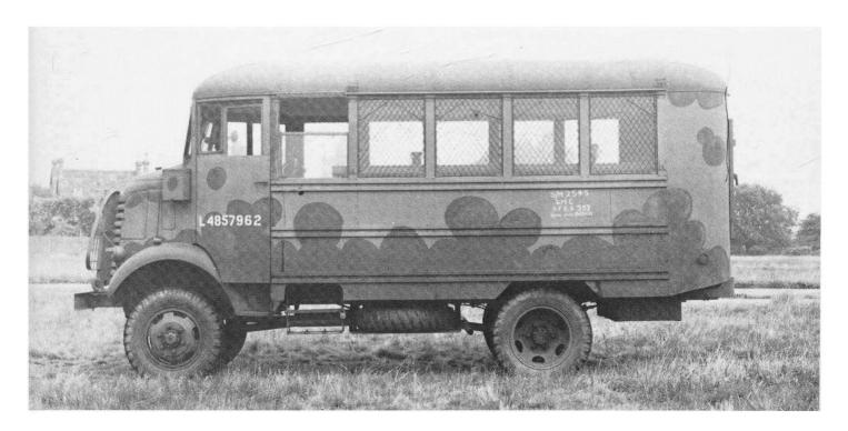
the British and Canadians, it was carried on  $15 \, \mathrm{cwt} \, 4 \times 2$  or  $4 \times 4$  chassis. The welding equipment was of the 300 amp electric type, powered by a separate engine and it made available the usual welding equipment such as a vice, table, welders screen and portable grinder together with a selection of electrodes for both normal steel and armour plate welding.
