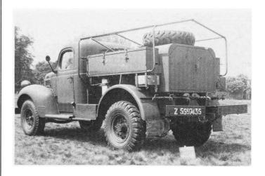
The Canadian-built Dodge D15, 15 cwt,  $4 \times 2$ , 200 gallon water tanker was also fitted with a CMP 15 cwt GS body and used by the British Army in large numbers.
