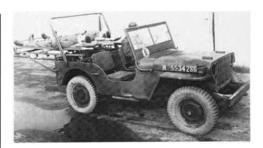
A Willys 'Jeep' fitted with British-designed two stretcher modification. An extended canvas hood was fitted to protect the casualties. Superseded by three-stretcher layout.
