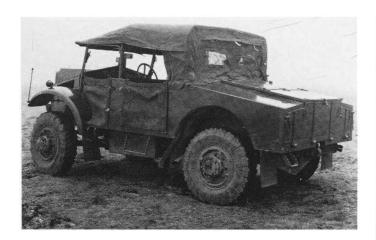
Morris 'Quad' prototype of  $4 \times 4$  field artillery tractor with open body.
