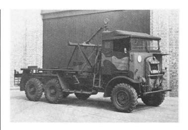
This was the final version of the Retriever with full screen, revised 'Thornycroft' type radiator, and raised cab sides. The body was to transport trackway-bridging equipment, and the front bumper was part of the bridge-laying gear.
