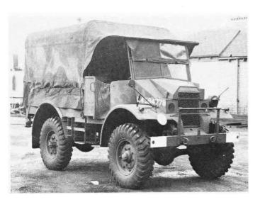
With the demise of the 2 pdr A/Tk gun many portees were converted to 17 pdr A/Tk gun tractors. This is a converted Chevrolet CGT.
