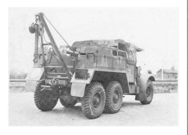
The Morris CD/SW 30 cwt light breakdown had a simple block & tackle hoist capable of lifting 1 ton. An example was used in early air-portability trials.
