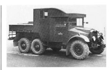
The prototype Morris CD/SW LAA tractor (census no. H 382455) with totally enclosed cab and gun crew compartment.
