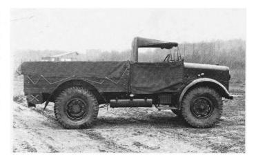
This shot of the prototype Bedford MW 15 cwt  $4 \times 2$  truck of 1937 should be compared with the production version, the bonnet slope being made pronounced.
