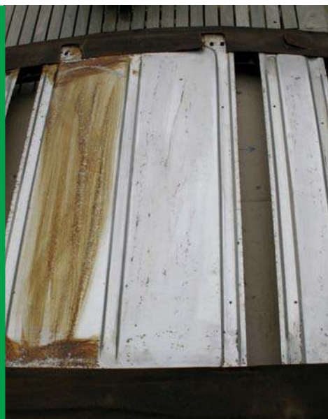
Roof plates from the top show how the webbing spaces them so the roof will fold. One half has had the old glue scraped off with a soft wire brush
