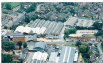
The haphazard layout of the old Newport Pagnell site shows why Aston Martin needed a new factory
