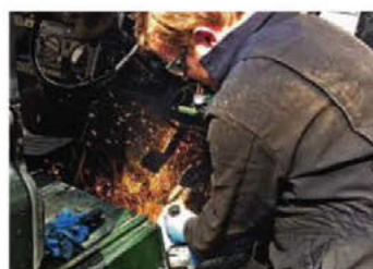
Grinder was needed to shift floor fixings
