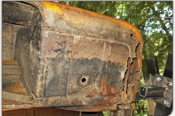
With substantial holes in the floor and no suitable reproduction or used panels to weld in, the restorers had to fabricate appropriate pieces to complete the body. Reproduction side panels, however, were available from his company, Clark's Corvair Parts.
