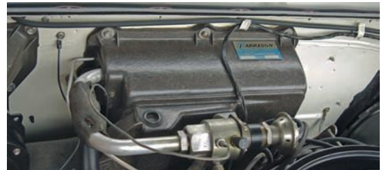
Even after more than 50 years, the Harrison A/C unit still looks brand-new, as if it were just installed.
