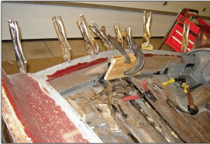
A few metal repairs needed to be made to the rear fascia as well. Several clamps were used to temporarily secure small patch panels before each piece was tack-welded. Again, seams were welded shut one small section at a time to avoid warping the panels.
