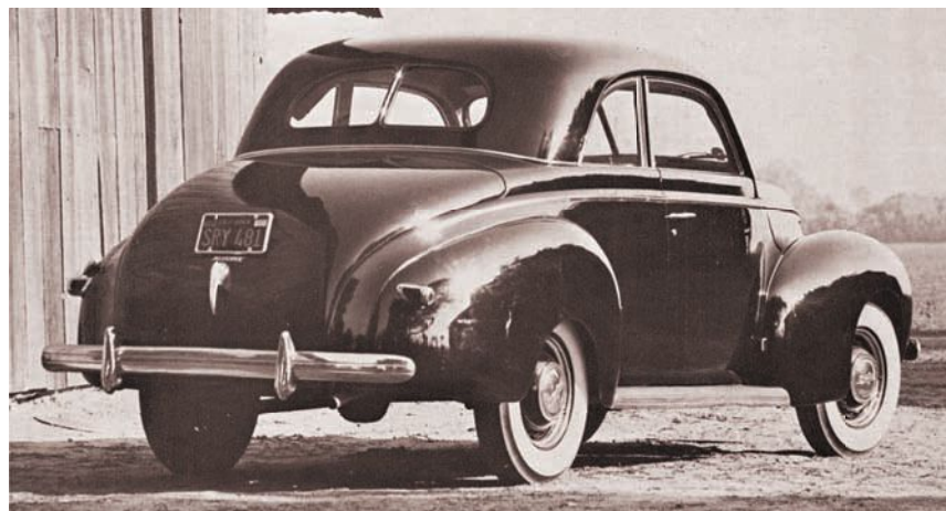
The most radically different body style was the sedan-coupe, which used convertible doors and very thin, chromed window surrounds.
