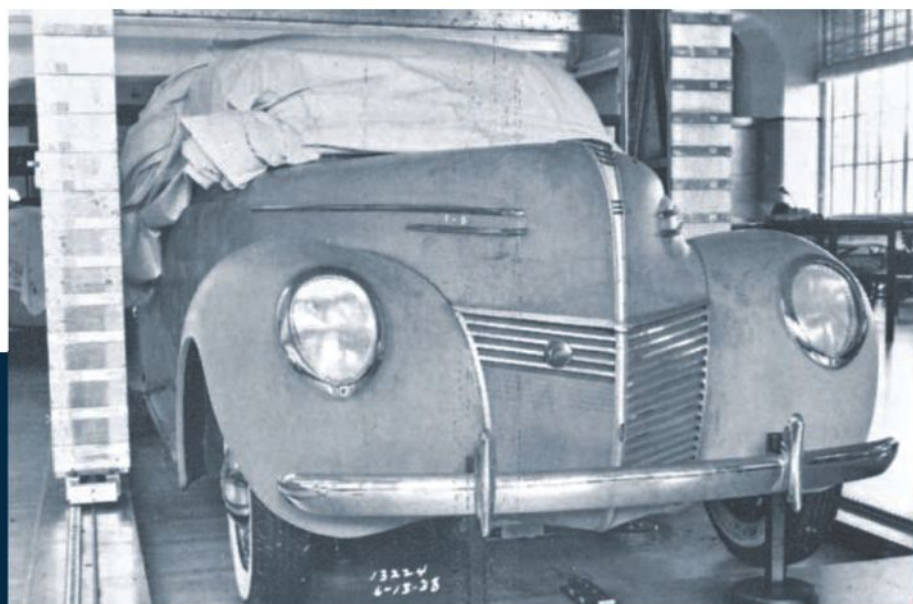
Front end takes shape by June 1938, but grille still says "Ford-Mercury," and bumpers aren't grooved. Original prototypes were built on extended Ford frames.
