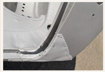
To prevent the body from flash-rusting, the bare metal was given a quick coat of protective self-etching primer. There were several other small pop-riveted patch panels exposed during media blasting, including the lower corner of the tail panel.
