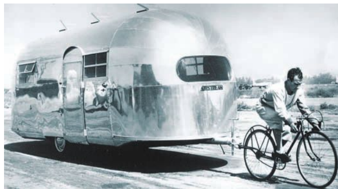
Just how light is an Airstream? Byam arranged for an expert bicyclist to demonstrate how light by towing it single-handedly with his bicycle.
