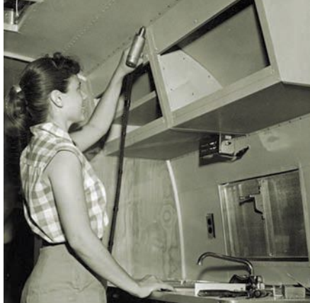
As demonstrated here, Airstream cabinets were riveted in place rather than screwed, for a better, longer lasting fit.
