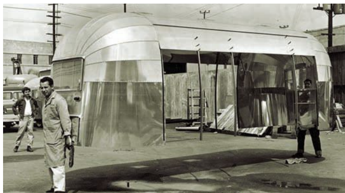
Mated to the rugged Airstream frame was an aluminum alloy body so light that two men could carry it easily.
