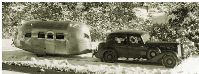
A 1938 Clipper in all its glory, being towed behind what appears to be a Packard. Airstream boasted fully insulated bodies and propane heat, allowing owners to use them in the winter.
