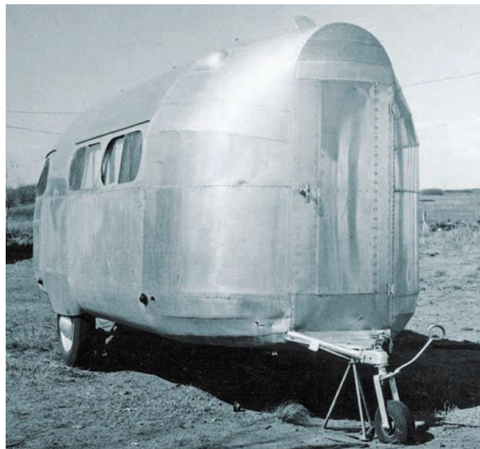
The 1935 Bowlus-Teller Road Chief, the trailer that became the template for future Airstreams. One drawback of the Road Chief was its front-mounted door, which restricted floor plan options. For Airstream, Wally Byam relocated the door to the side.
