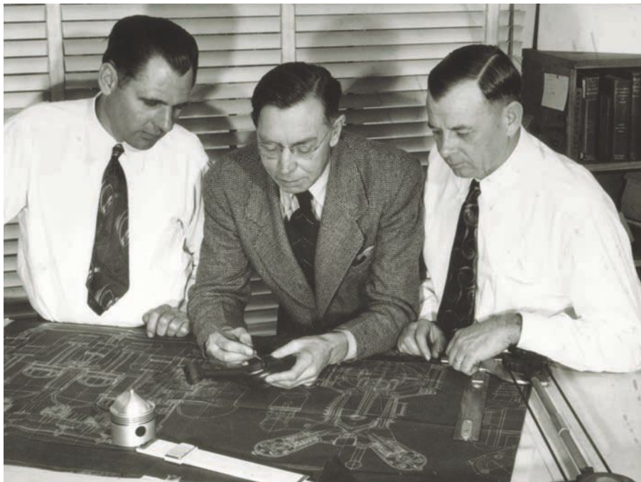
Fred Offenhauser's successors: From left, Louis Meyer, Goossen and Dale Drake at the drafting table, 1947. Goossen's drawing shows the "pentroof" design of the original 220 Offy.
