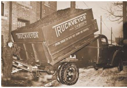
coal box so the chute could have a steeper angle. The elevated box either had the dump feature or else it had a steeply sloped floor, which fed the coal through a door in the bottom of the center.
