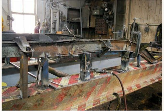
Next was the fabrication of new body mounts to replace the originals that had corroded away over time. These were critical, and making them now would save time later in the process. Note that a small side rail has been welded in place to help maintain frame width later.
