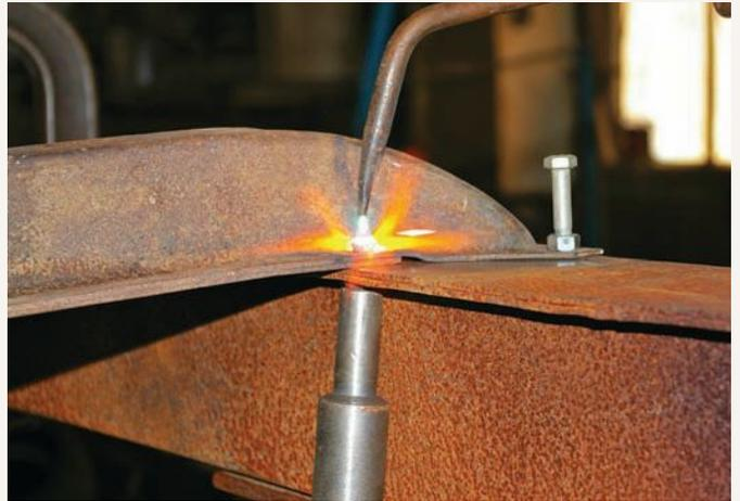
Since André wanted to maintain as many factory-built aspects as possible, he opted to reassemble the frame using rivets rather than modern bolts. With a new rivet positioned from below, heat was concentrated on the butt end and then hammered closed.
