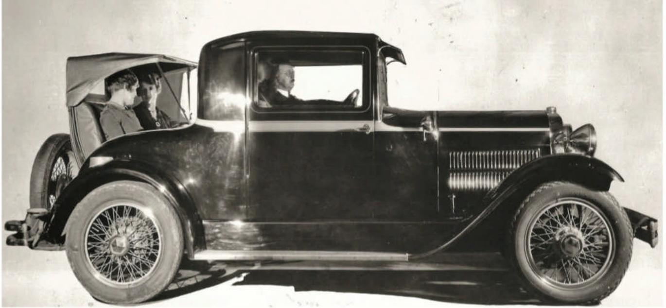
In 1929, Hudson's designers came up with a neat, though rarely seen, option for rumble seat coupes and roadsters. Called the "Rumble Roof," it provided passengers in the rumble seat with a degree of protection from the elements.
