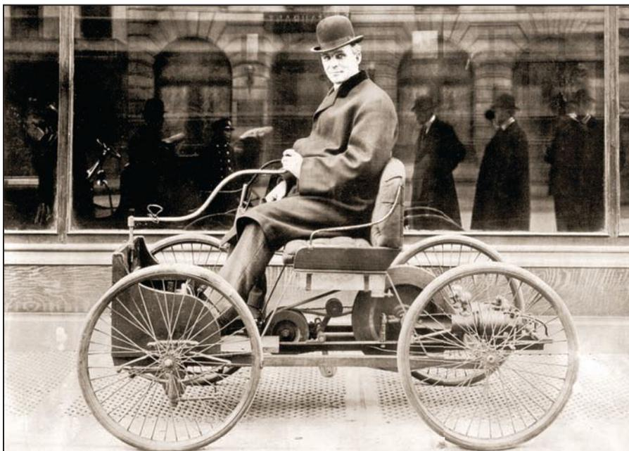
**HENRY FORD'S QUADRICYCLE RUNS ON FOUR BICYCLE WHEELS AND A TWO-CYLINDER,** rear-mounted engine capable of propelling the vehicle at around 20 miles per hour. Ford debuted the Quadricycle on June 4, 1896, and it was indeed able to attain the 20-mile-per-hour mark. The 32-year-old inventor intends to make more Quadricycles in the future.
