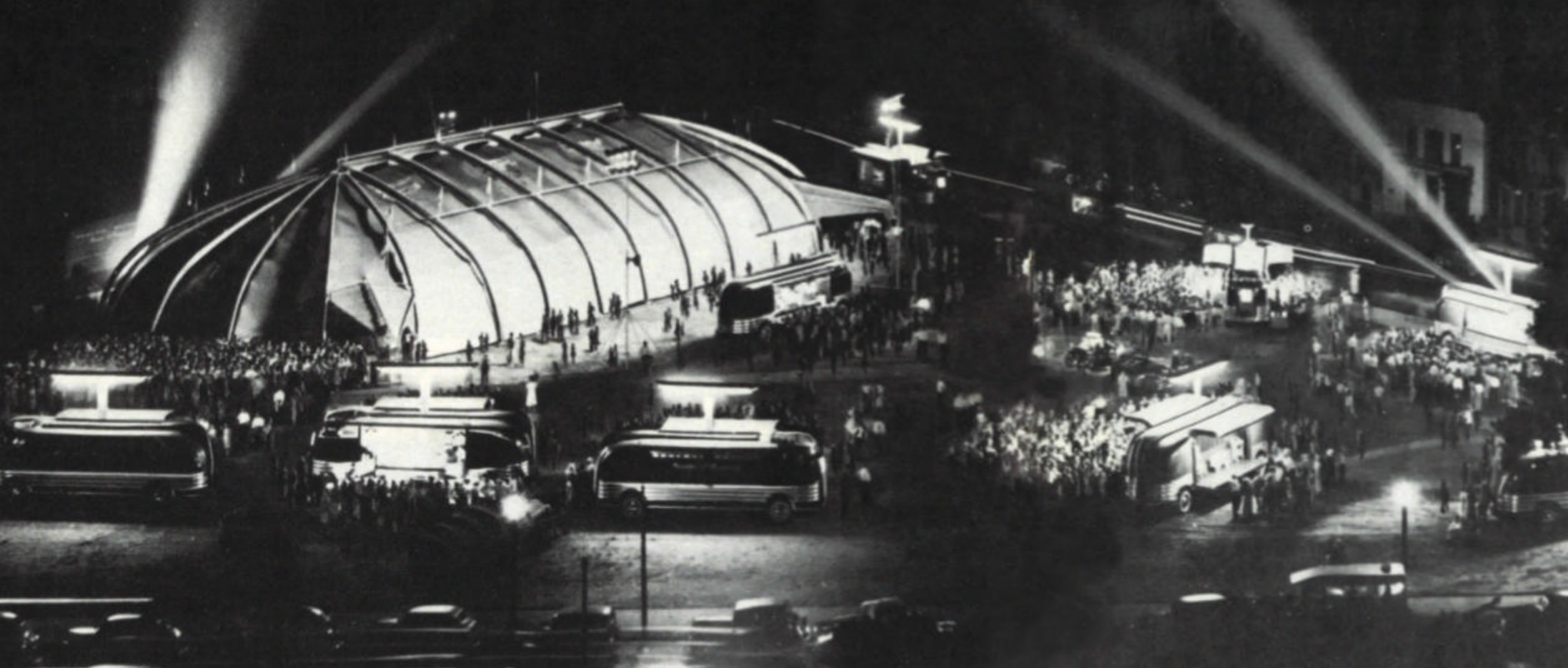
After 1940, the Parade used a tent invented by Fred Huddle, with collapsible aluminum exterior girders and aluminized canvas. Free shows attracted many millions of people and gave GM fine publicity.
