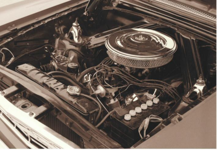
ABOVE: The 260 Sprint engine for 1964 featured chromed accents, but in the production models the chromed tops of the shock mounts shown in this factory photo were painted, the air cleaner was different, and the battery was on the opposite side. BELOW: The 170-cu.in. straight-six engine was rated at 101 hp in 1964 and 105 hp in 1965. Note "Falcon Show Car X-511-2" written on the cowl-to-shock-tower brace of this 1965 model.
