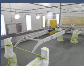
The simple, sturdy frame was repaired and refinished as the deceptively simple foundation for rebuilding the Springfield Rolls.
