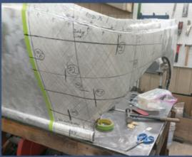
Metal fabrication, along with re-wooding, are core skills at LaVine Restorations, so creating templates and replicating the undamaged portions of the body in mirror image were relatively straightforward processes.
