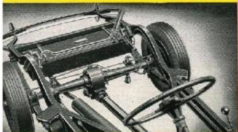
The front drive is taken by a floating underslung worm and wheel rear axle. Note the long semi-elliptic springs, robust chassis frame, built-in jacks and anti-roll torsion bar.
