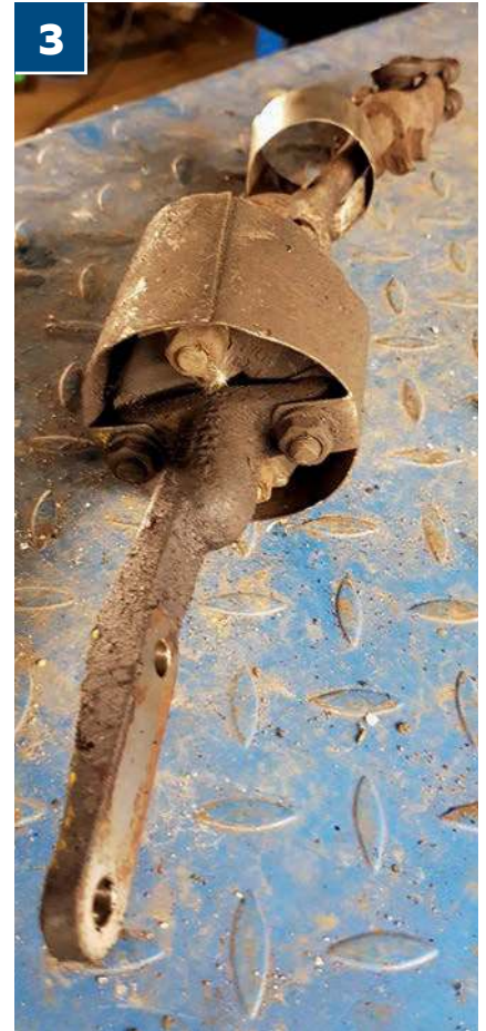
3 Down below, steering components needed to be removed to allow enough space to drop the same manifold from where it has been sitting for the past four decades
