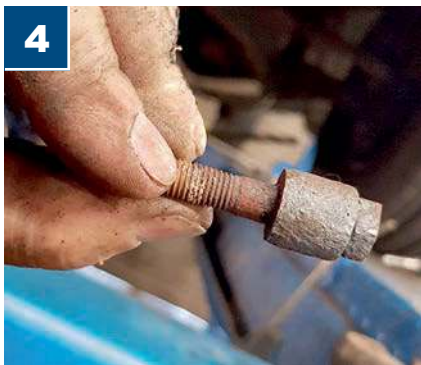
4 Some of the bolts were stuck fast, while some were only finger tight – but most bolts put up a fight, refusing to come loose and remaining seized into their collars
