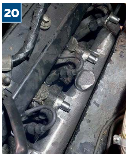
20 With the obstructing hardware already removed, the new offside manifold, its gaskets, bolts and joint collars were fastened into place
