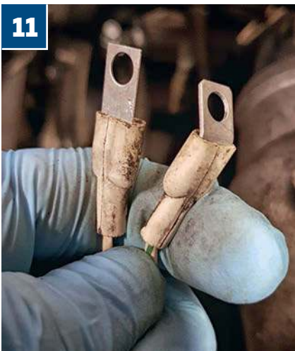
...and here are two of them fitted to the car's ignition coil wiring
