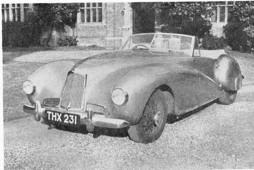
DB1: The 1948 Aston Martin drophead coupé, with 2-litre four-cylinder engine, first of the very successful DB series of post-war Aston Martins.
